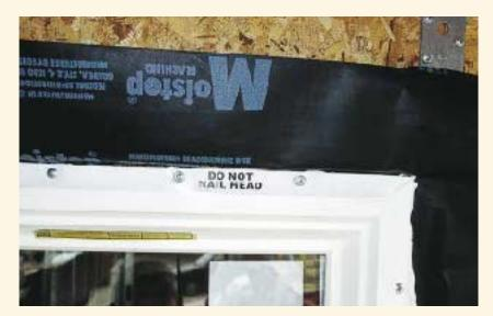
**Figure 4.** Comparing installation instructions from different vinyl window manufacturers reveals a jumble of contradictions. For example, some recommend attaching the fin at the top of the window, while others warn against it. The conflicting advice causes many installers — including the one who installed this window — to risk voiding the warranty by ignoring the manufacturer's instructions.
