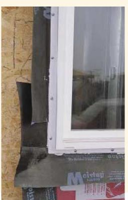
Figure 5. Flexible flashing at the side of the rough opening should extend over the flashing at the bottom. Here, the side flashing was cut too short, and the installer incorrectly failed to lap the filler piece over the bottom flashing. When housewrap or felt paper is later installed, it should be tucked under the horizontal flashing at the bottom of the window.
