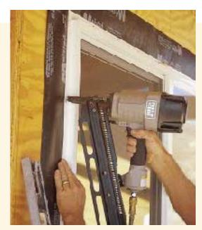
**Figure 6.** The use of nail guns is discouraged by some manufacturers, who prefer to see the fasteners left proud to allow for window movement. Also be careful to avoid driving additional nails into the nailing fins when installing trim and siding.
