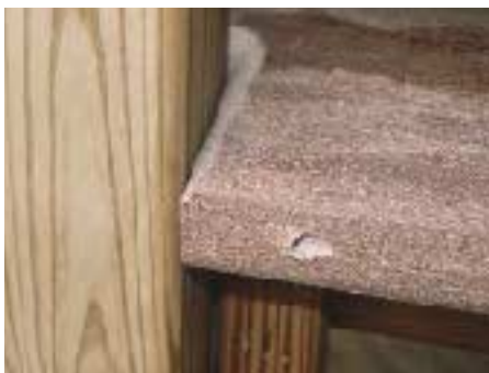
Figure 8. Simple, router-rolled corners finish nearly every edge and joint in the system, giving an appearance of heightened detail while concealing small deviations in plane and material thickness.
