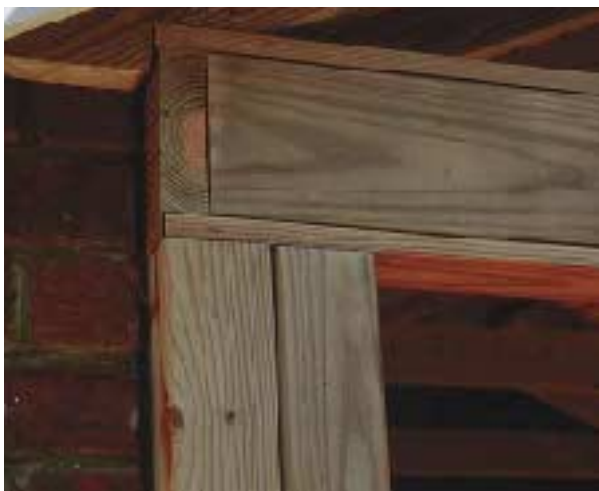
Figure 3. A box beam lintel consisting of 1x4 plates and 2x6 sides caps the 4x4 posts and runs the entire perimeter of the porch enclosure.
