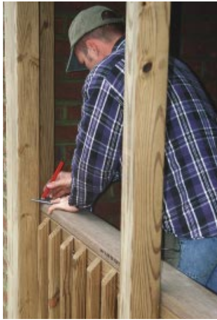
Figure 5. Surface-installed rails and balusters simplify construction and protect the screening from damage by children and pets. Because the screening doesn't contact the railing or balusters, they are barely visible from outside.
