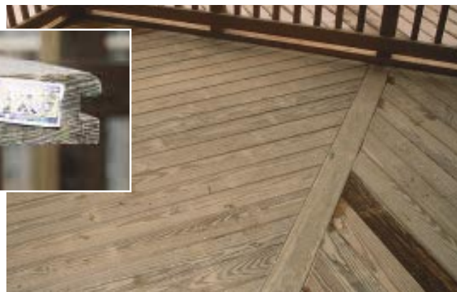
Figure 1. The author installs 2x6 pressure-treated T&G decking to prevent insects from entering between the floorboards of a screened porch. The decking is blind-nailed through the tongue to conceal the fasteners.
