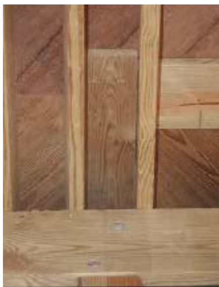
Figure 2. Two-by blocking, installed on the flat between joists, supports the transition between the diagonally installed porch and Trex sundeck surfaces.
