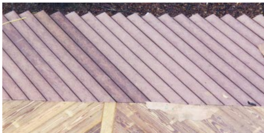
Figure 2. Two-by blocking, installed on the flat between joists, supports the transition between the diagonally installed porch and Trex sundeck surfaces.
