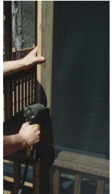
Figure 6. Asphalt roofing staples hold the screening tight, and are less tiring to install than conventional screen staples. Sagging screen is pulled tight between staples and secured to ensure a drum-tight fabric installation.
