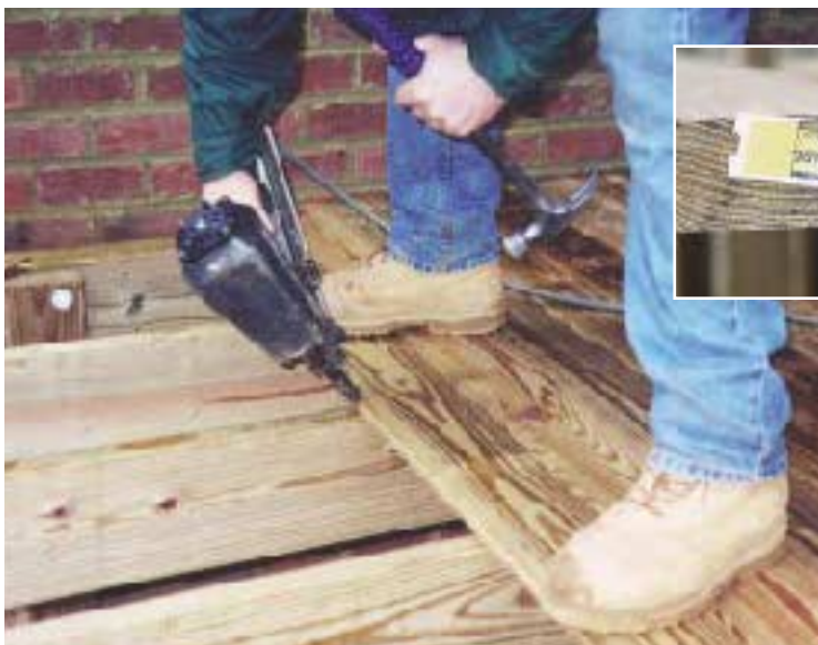
Figure 1. The author installs 2x6 pressure-treated T&G decking to prevent insects from entering between the floorboards of a screened porch. The decking is blind-nailed through the tongue to conceal the fasteners.
