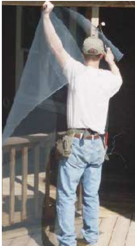
Figure 6. Asphalt roofing staples hold the screening tight, and are less tiring to install than conventional screen staples. Sagging screen is pulled tight between staples and secured to ensure a drum-tight fabric installation.
