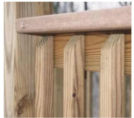
Figure 5. Surface-installed rails and balusters simplify construction and protect the screening from damage by children and pets. Because the screening doesn't contact the railing or balusters, they are barely visible from outside.
