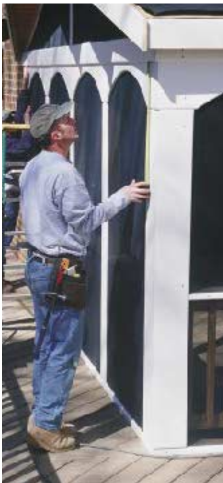
Figure 7. The author uses a simple method for producing custom arches in the continuous, dropped headcasing that accents the individual screen openings. After establishing the radius point of the arch, he uses a site-made trammel stick to draw it directly on the 1x12 stock. The resulting arch, cut with a jigsaw, is perfectly matched to each opening.
