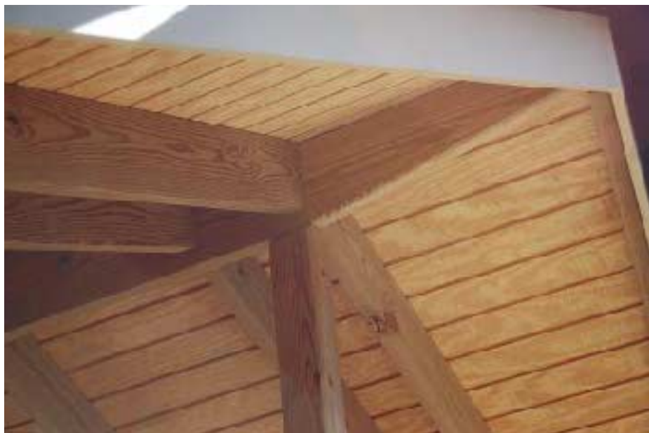
Figure 4. The author's signature "flying gable" roof helps keep windblown rain out of the porch.
