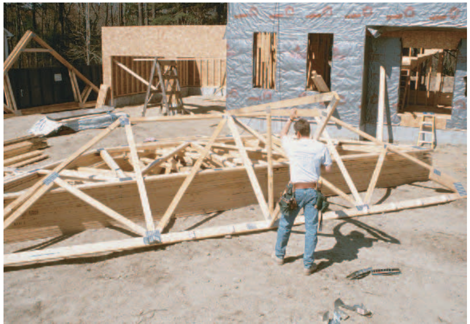
Figure 4. A single jack truss nailed to the girder truss will hold it upright while the rest of the jack trusses are installed.
