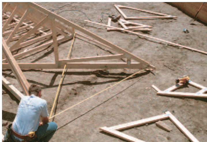
Figure 10. Before installing the corner jack trusses, it's important to recheck the position of the end of the girder truss and the hip truss.
