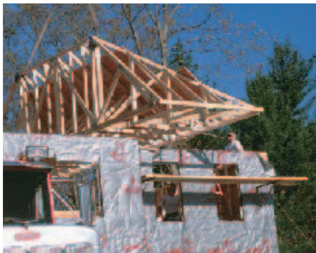
Figure 15. The truss assembly is easier to control if it flies level. Secondary straps extending to the subfascia can be used to help level the trusses during the lift.
