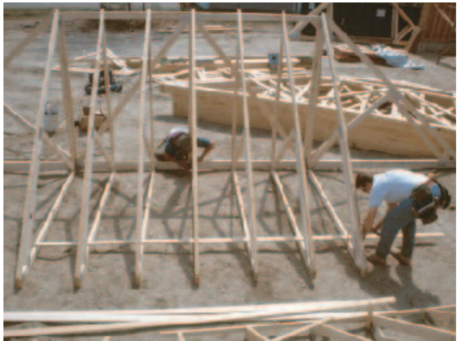
Figure 5. Once the jack trusses are fastened to the girder, a long 1x3 holds the tails of the jacks in position.
