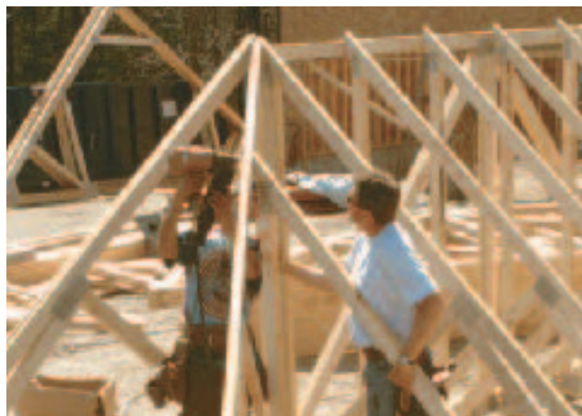
Figure 11. It's handy to have two people to help position the corner jacks on the hip trusses. The corner jacks are nailed at the top through the top chord of the hip truss.
