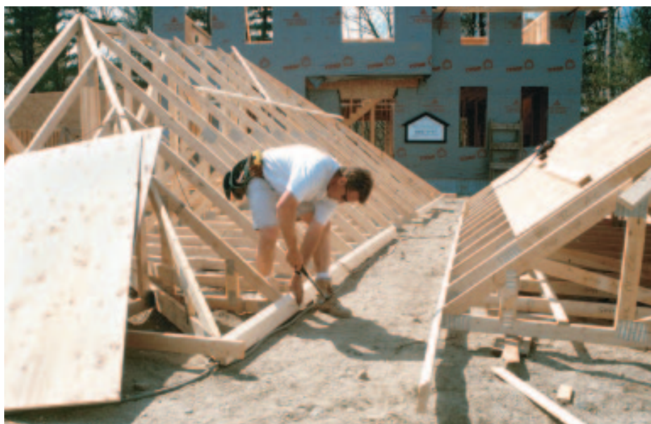
Figure 13. A subfascia ties the tails of the trusses together and stabilizes the truss assembly for lifting.
