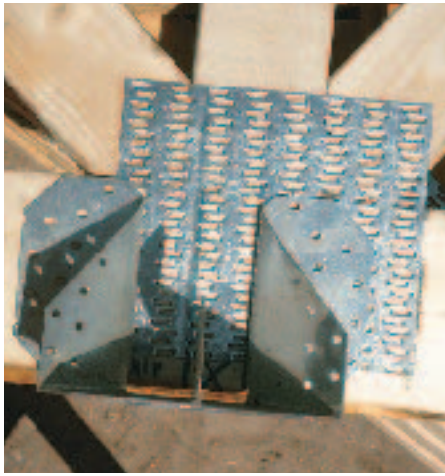
Figure 3. This universal hanger supports both the hip truss and one of the jack trusses. This type of hanger is reversible and can be used on either the left or the right side.
