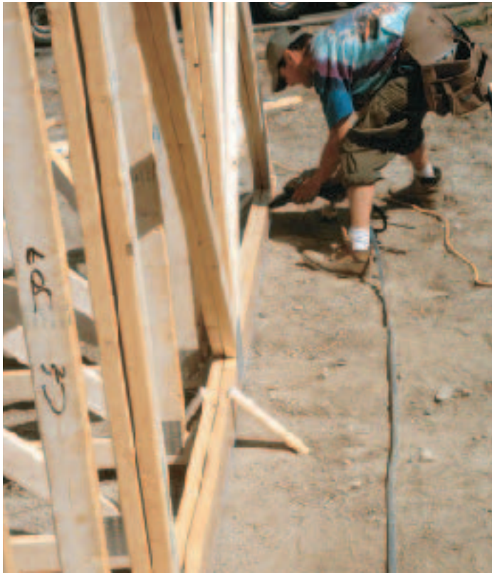
Figure 8. The second girder truss is paired with the first after the jack trusses and hip trusses have been installed. Before the two girder trusses are nailed together, they have to be straightened to a string. Diagonal 1x3s and kickers driven into the dirt are used to persuade the girder into position.
