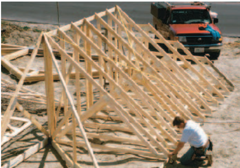
Figure 7. The jack trusses are squared to the girder truss by checking the diagonals across the top chords.
