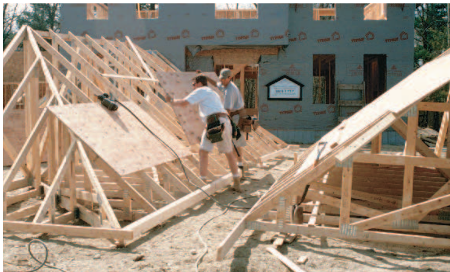
Figure 14. To facilitate fastening the trusses to the wall plates, the bottom course of sheathing can either be nailed loosely or be omitted.
