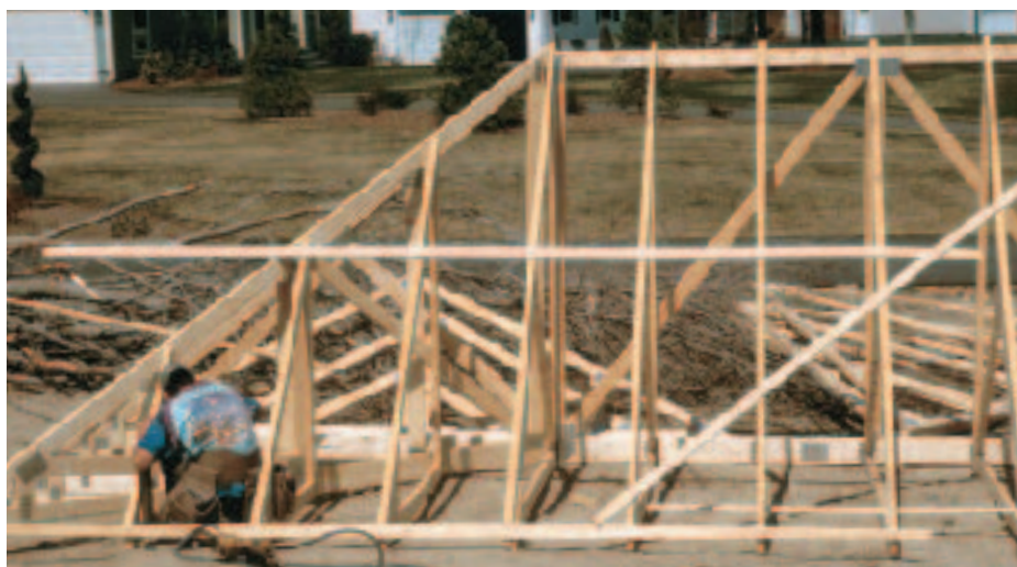
Figure 12. To hold the tails of the corner jacks at 24 inches on-center, they're nailed to the 1x3 that was used to position the hip.
