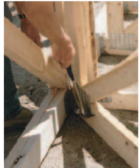
Figure 9. Once the two girder trusses are nailed together, the rest of the hanger nails can be installed.
