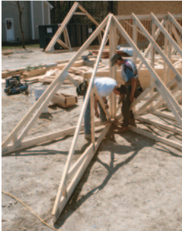
Figure 6. The hip truss is installed tight to the corner where the outside jack truss meets the girder truss. Although the vertical web in the corner should not be trimmed with a bevel, the tail of the hip truss needs to be trimmed on site with two 45-degree bevels.
