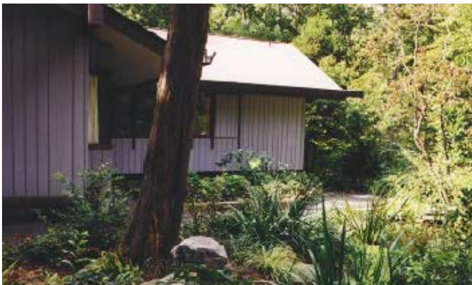
Figure 4. Eight weeks, 440 carpentry hours, and $25,000 later, the house — shown here the following summer — was at least as good as new.
