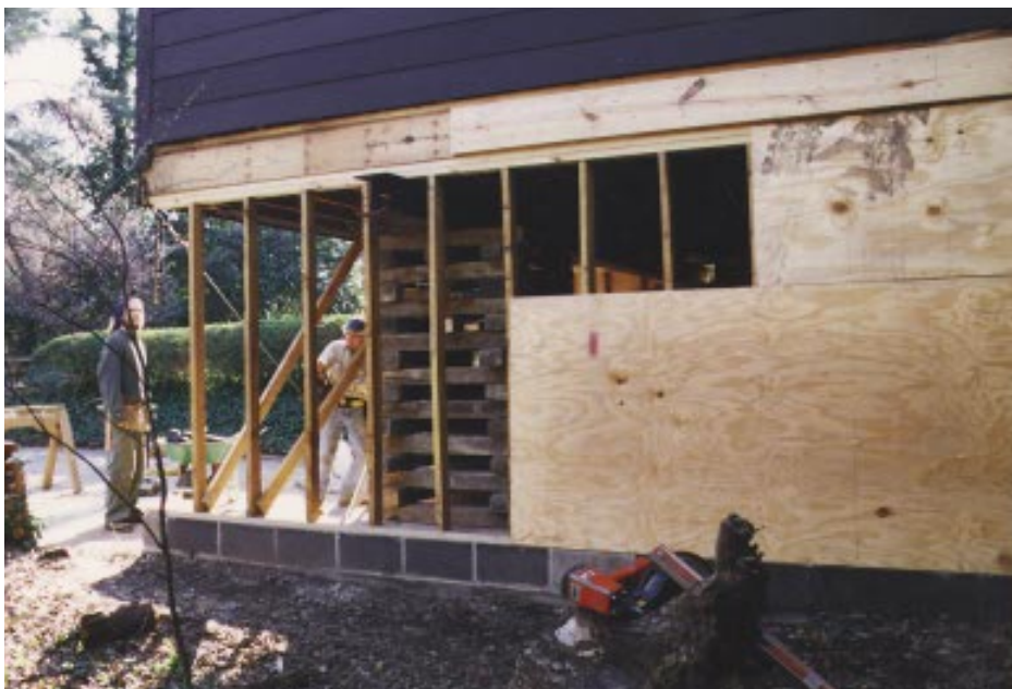
Figure 8. After some minor foundation repairs and the placement of new anchor bolts, new garage walls were framed and partially sheathed (above). At the last minute, the steel beams were eased out of their slots, shifting the second-story load onto the foundation (right).
