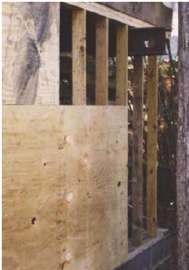
Figure 8. After some minor foundation repairs and the placement of new anchor bolts, new garage walls were framed and partially sheathed (above). At the last minute, the steel beams were eased out of their slots, shifting the second-story load onto the foundation (right).
