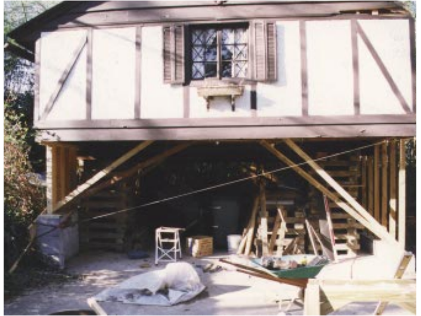
Figure 9. To square up the garage door opening, the completed frame was carefully racked with a come-along (left), and the temporary diagonal bracing shown above was replaced with shorter, permanent braces.
