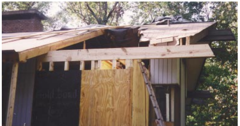
Figure 3. Replacing the cantilevered beams that supported the gable-end overhang was a time-consuming task that called for some discussion with the homeowner's insurance adjuster.
