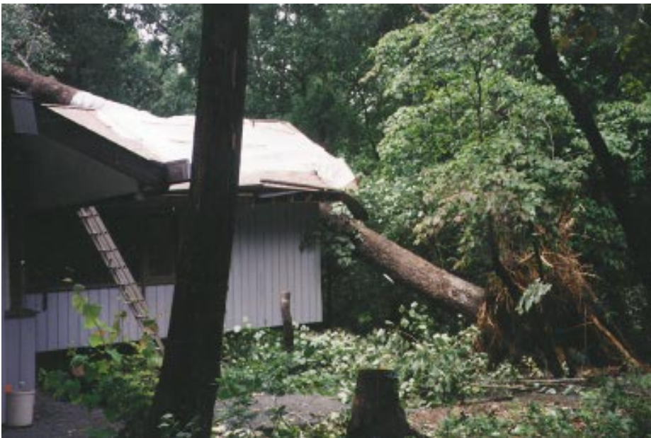
Figure 1. Felled by a September hurricane that veered inland, this mature poplar tree was an unwelcome house guest (right). The first order of business was to cover the gaping hole — and the tree within — with 6-mil plastic to keep out the rain (below).
