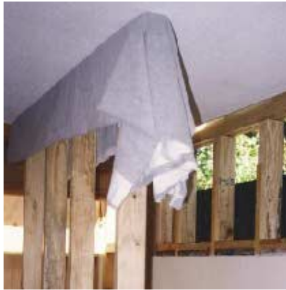
Figure 2. The undamaged bedroom ceiling was braced with a temporary wall cushioned by a folded drop cloth (left). Broken framing members like this 4x10 beam (below) were cut back to sound wood.
