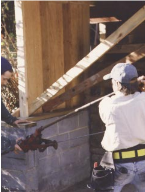
Figure 9. To square up the garage door opening, the completed frame was carefully racked with a come-along (left), and the temporary diagonal bracing shown above was replaced with shorter, permanent braces.
