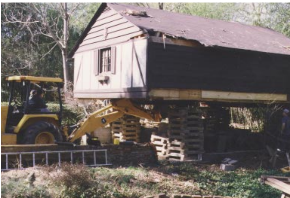
Figure 7. Once elevated on cribbing (top), the structure was carefully repositioned with a backhoe, aided by small steel rollers placed beneath the supporting steel I-beams (bottom).
