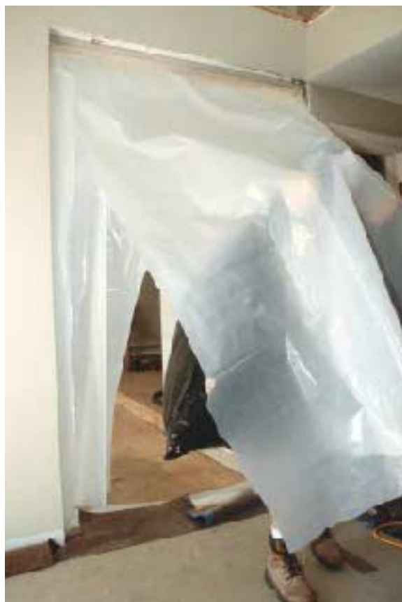
Figure 3. The "tee lock" that serves as the main entrance to the work area starts as a double layer of poly stretched across a doorway. The outer layer is then cut loose on the sides and bottom, forming a flap. The inner layer is slit across the bottom and up the center, in the shape of an upside-down letter T. It admits needed makeup air when the air handler is operating but not so much that the work area loses its negative pressure.
