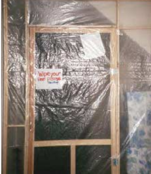
Figure 4. A poly-covered screen door on spring-loaded hinges can be useful if the homeowner has to pass through the work area during off hours. The poly should be applied to the living-space side of the partition, so air pressure sucks it inward against the framing.
