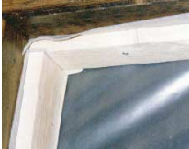
Figure 1. The work area is separated from the job site with site-built partitions of 1x3s and 6-mil poly. Closed-cell foam sill sealer between the strapping and door jamb provides a good seal.
