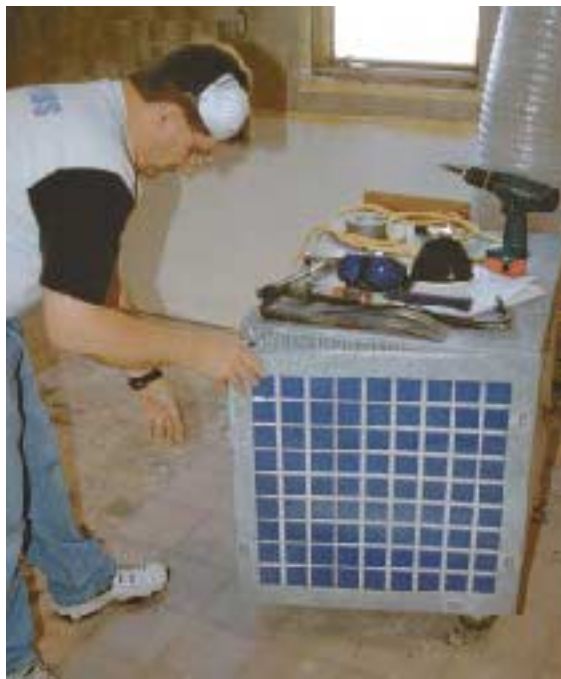
Figure 5. A 2,000-cfm air handler (near right) keeps the work area under constant negative pressure to prevent dust from escaping. The filtered exhaust air is vented through a 12-inch mylar hose (middle), which is securely taped to a plywood panel mounted in an open window. Besides reducing the lead hazard, the air handler makes demo work much less uncomfortable. The layer of dust on the air handler prefilter (far right) represents an hour's worth of tearing down ceiling drywall backed with blown fiberglass. In an unventilated area, most of that would be clogging the air.
