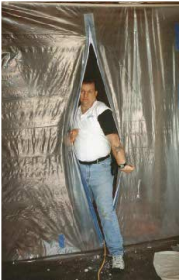
Figure 2. Self-adhesive zipper doors are easily applied to poly partitions, providing access while maintaining negative pressure in the work area. Minor holes in the poly partition can be repaired with tape.
