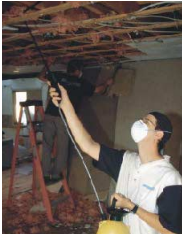
Figure 6. Drywall, plaster, and other dusty materials are misted with water before removal to keep airborne dust to a minimum. Material on the floor is misted again before being shoveled into bags for disposal.
