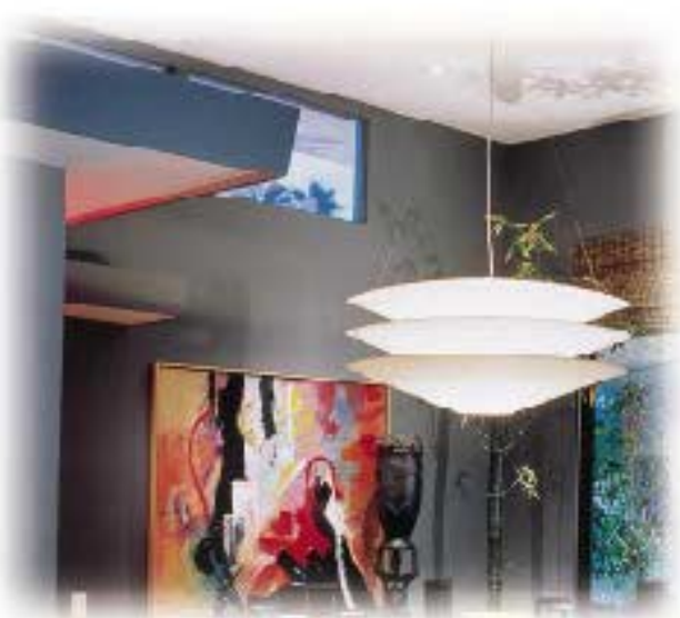
Figure 8. The pendant fixture in this dining room directs most of its light toward the ceiling. The light from the pendant is balanced with ambient cove light and accent light on the painting.
