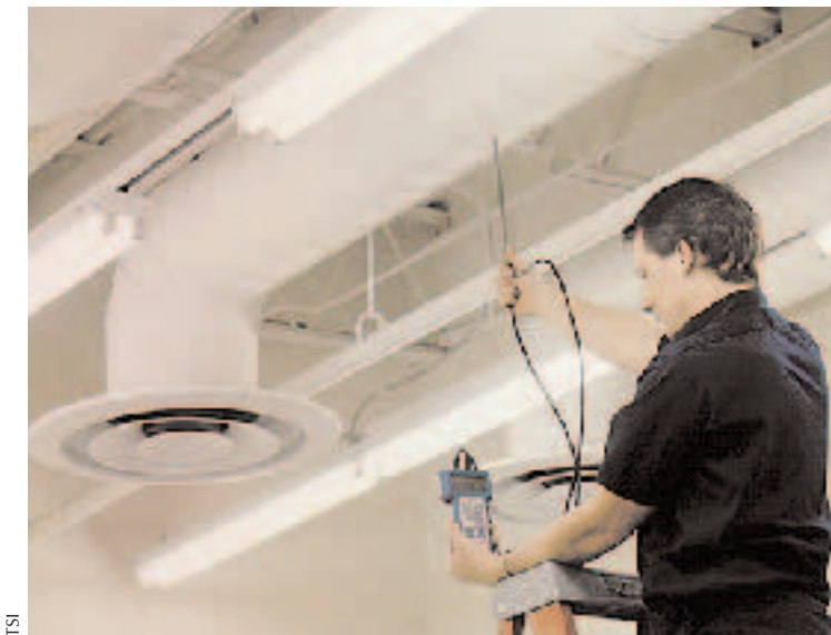
Figure 5. Static pressure can be measured with a simple magnehelic gauge or with a sophisticated digital manometer like the DP-Calc from TSI, shown here.
