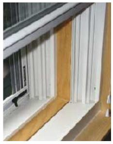
**Figure 10.** Even the windows get doubled in a sound-insulated room. Thermopane glass, minimum 2-inch air spaces between units, and a high-performance storm window present an effective barrier to external noise.
