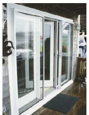
Figure 3. Sliding storm panels provide extra sound insulation at sliding door locations. In every instance of a secondary door or window, there should be a minimum 2-inch gap between primary and storm units.
