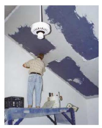
**Figure 7.** Applying the principle that surface mass absorbs noise energy, adding an extra <sup>5</sup>/8-inchthick layer of gypsum blueboard with a plaster skim coat helps to reduce the noise transmitted through flat-roof and cathedral-style ceilings.
