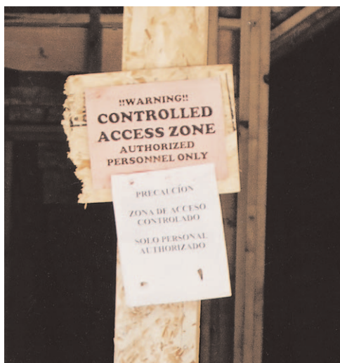
Figure 1. The first step in conforming with OSHA's alternative fall protection method is to establish a job site Controlled Access Zone and see that it's enforced.
