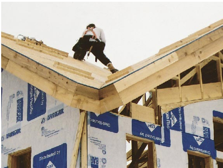
Figure 5. Spacing of slide guards is determined by roof pitch. Regardless of spacing, though, individual guards must be at least a nominal 2x4 on edge, set perpendicular to the slope.
