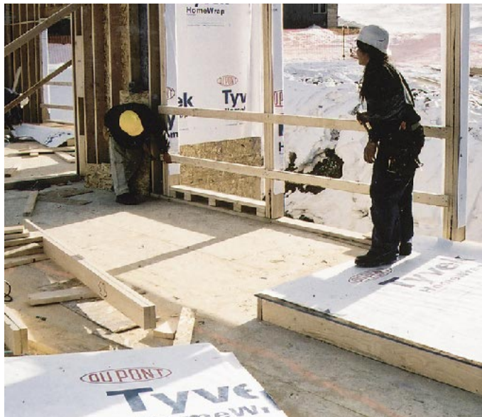
Figure 2. A painted warning line 6 feet from the edge of the second-floor deck is an acceptable substitute for guard rails until the walls have been framed and erected. At that point, it’s necessary to install guardrails where needed, as shown here.
