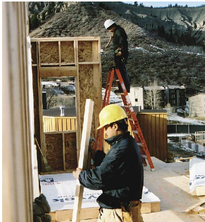
Figure 3. No more walking on the plate. Wall plates must be tied together from ladders or scaffolds.
