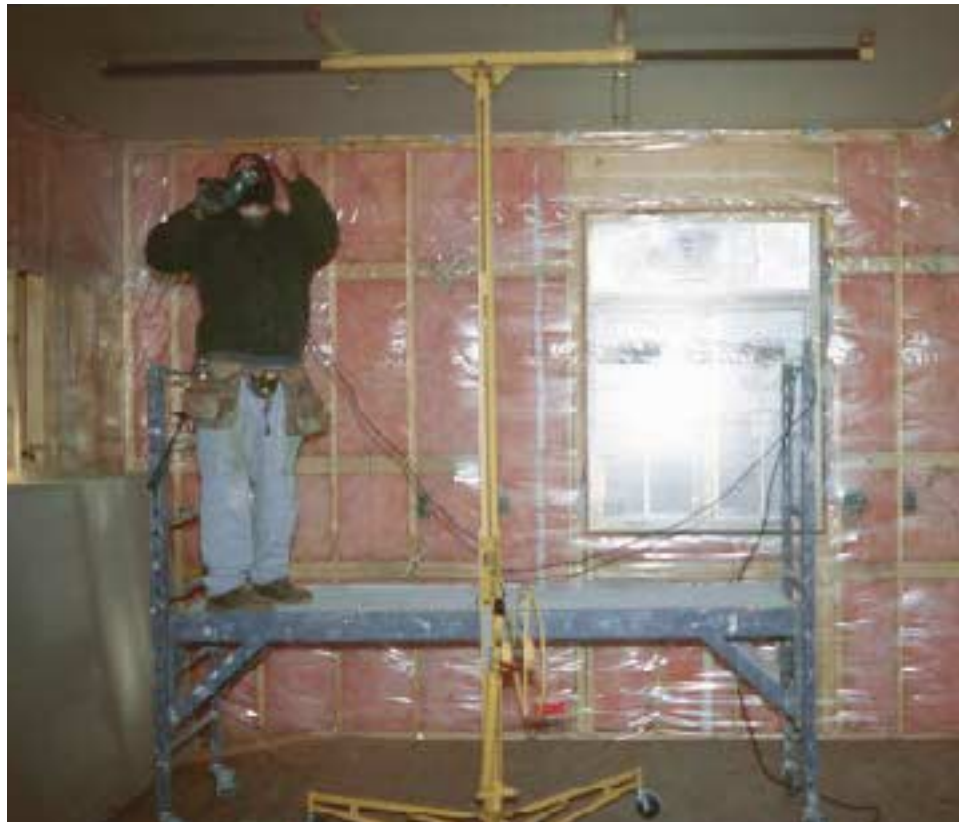
Figure 4. A baker's scaffold rolls easily through doorways to provide a mobile platform for ceiling work up to 12 feet high.
