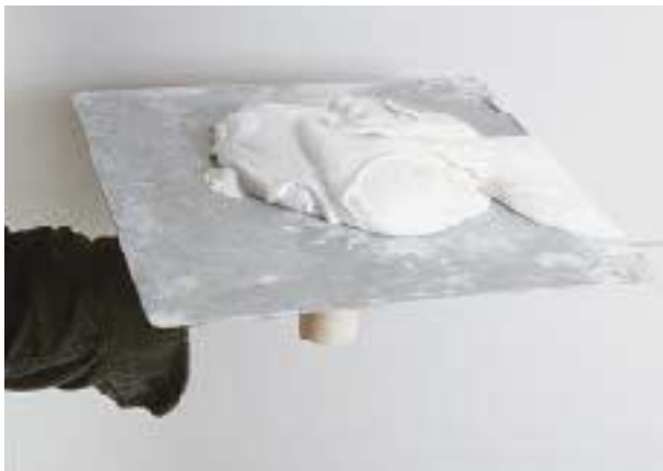
Figure 11. Thinned compound will slide off a hawk (left), but stays contained in a mud pan (below).
