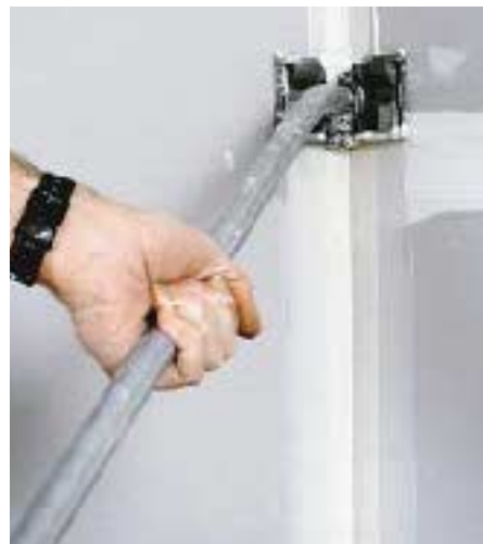
Figure 18. A corner roller embeds tape in the compound following its application by the automatic taper (far left). An angle applicator attaches to the corner finisher to deliver compound to the surface for tooling. The 3-inch adjustable corner finisher smooths and feathers the compound after the tape is embedded by the corner roller (left).
