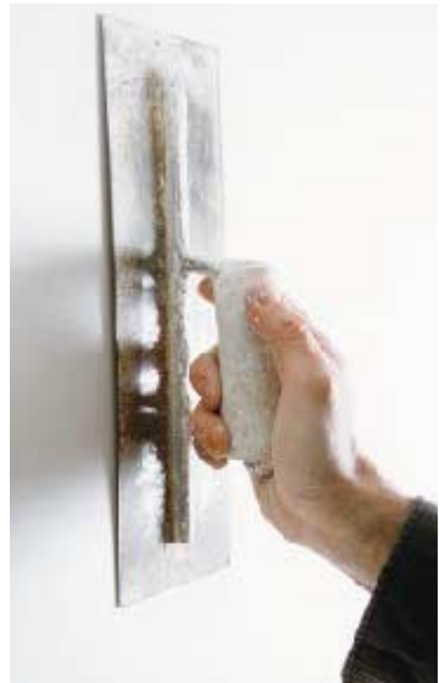
Figure 10. A curved-blade trowel puts a perfect crown on finished joints and creates great feather edges.
