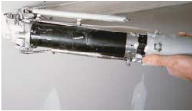
Figure 16. An automatic taper applies paper tape and compound simultaneously to seams and corners.
