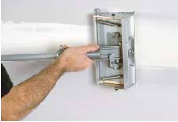
Figure 19. A flat box dispenses second and third coats to the taped joints. An adjustable curve in the blade ensures a precise, feathered crown on flat seams.
