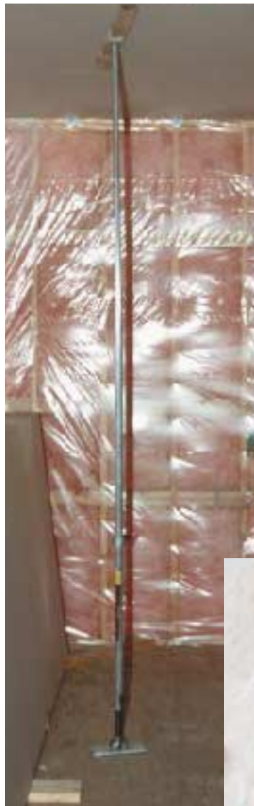
Figure 5. The adjustable, locking Stiff Arm deadman provides temporary overhead support when hanging ceiling panels.
