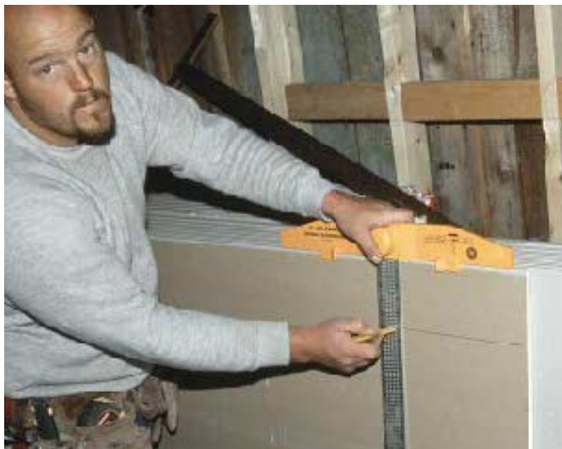
Figure 1. This pro-duty T-square from Warner has a 1/4-inch-thick tongue (left); most lumberyard varieties have only 1/8-inch-thick tongues. Graduated notches on the Johnson 24-inch ripping square guide make it easy to use a utility knife for long cuts (above).
