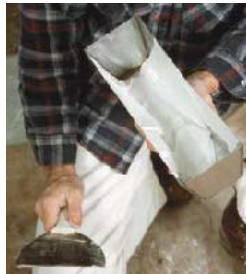
Figure 11. Thinned compound will slide off a hawk (left), but stays contained in a mud pan (below).
