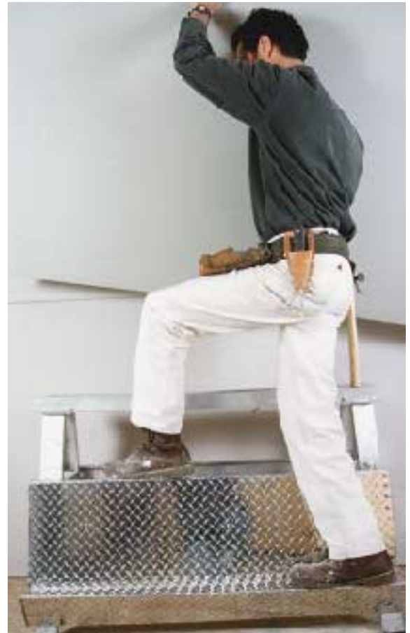
Figure 3. An adjustable aluminum drywall bench provides enough elevation to hang ceilings up to 10 feet high. At the highest adjustment, a detachable "Mack's Step" accessory adds an intermediate step and more stability.
