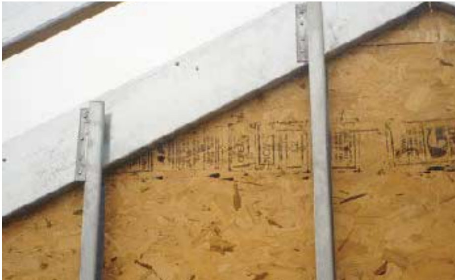
Figure 3. Gable-end studs are notched and bent to form attachment flanges before being screwed to the end rafters (left). Note the green layout line on the stud, drawn with a permanent marker before the flange is formed with duckbill locking pliers (right).
