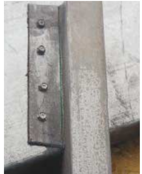
Figure 3. Gable-end studs are notched and bent to form attachment flanges before being screwed to the end rafters (left). Note the green layout line on the stud, drawn with a permanent marker before the flange is formed with duckbill locking pliers (right).
