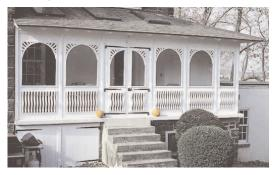
The panels are available in three trimmable widths (3, 4, and 5 feet). Each panel is divided horizontally by a rail into a large upper opening and a smaller lower opening, which can be ordered with balusters or solid panels if desired. All of the panel rails are reinforced with concealed steel rods. The aluminum-framed screens and tempered glass panels are secured to the cedar frames with clips.
