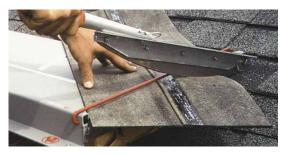
a "table" keeps the tool steady and anchored when working on a staging plank. The aluminum tool itself is light (18 lb.), making it easy to carry up a ladder.
