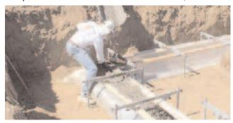
2x4 "kickers," and *Fastfabric*. The adjustable Fast-Yokes and the 2x4s can be reused. Enough Fast-Yoke brackets for a 200-ft. foundation (30 Fast-Yokes) cost about \$2,000 US, while a standard bundle of Fastfabric (120 ft. long by 62 in. wide) costs about \$52.
