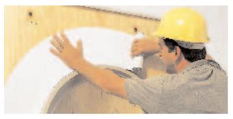
The membrane is made of butyl, not rubberized asphalt. The top layer is corrugated Tyvek, which protects the butyl from UV degradation during construction.
