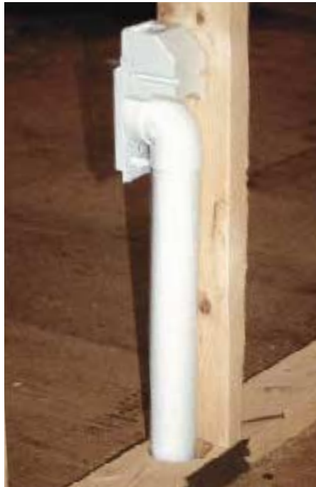
Figure 3. Short 90-degree ells are used at the inlet valve only. Full-sweep 90s elsewhere ensure unrestricted airflow in the system tubing.
