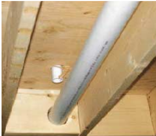
Figure 4. To avoid conflicts, central vac tubing is best installed after the electrician and the plumber have completed their rough-ins. Inlet valves can also then be mounted to match electrical box heights.
