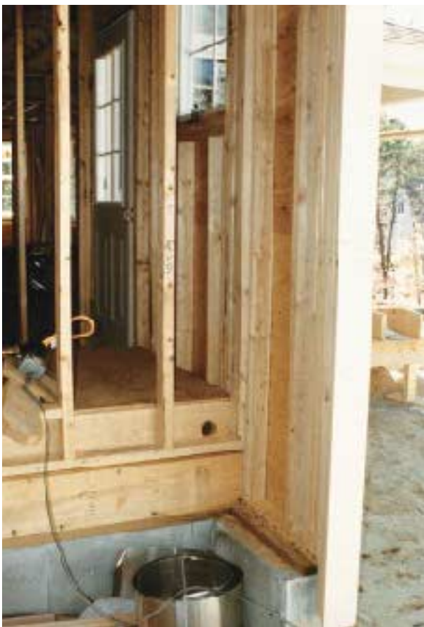
Figure 5. An inlet valve located close to the garage's overhead door eliminates the need to pull the car in for cleaning.
