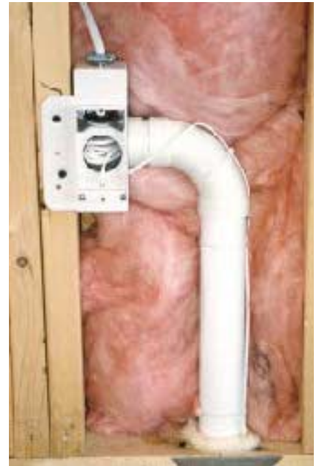
Figure 3. Short 90-degree ells are used at the inlet valve only. Full-sweep 90s elsewhere ensure unrestricted airflow in the system tubing.
