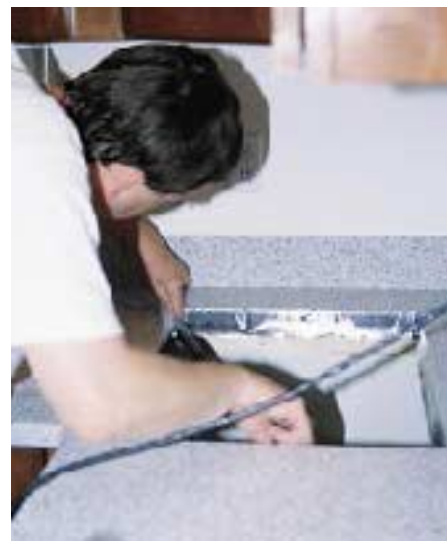
Figure 3. Two layers of special aluminum conductive tape, applied to the perimeter of a cooktop cutout, help deflect cooktop heat away from the solid-surfacing and into the supporting cabinet box.
