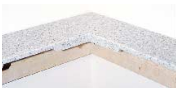
Figure 2. Square blocks of solid-surface material are glued to the underside of the counter (above) to reinforce the corners of the cutout (right).
