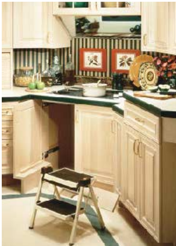
Figure 4. A contrasting color for the countertop edge provides an important visual aid for eyes with limited depth perception. Note the mirror mounted above the cooktop — no need to peer into a boiling pot to see what's cooking.
