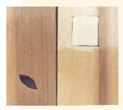
To provide needed contrast with the red cedar, cutouts in the design are backed with white cedar inlays (above). Williams air-nails the field shingles but reverts to hand-nailing for the fancy stuff (above, right). At right, the nearly completed figure.
