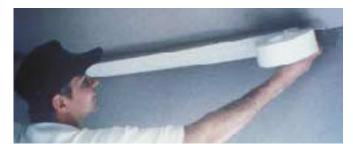
90-degree inside and outside corners, the flexible plastic tape can be applied using compound, staples, or the preferred proprietary spray adhesive. Edge-notches at 12-inch intervals make sizing easier. A 100-foot roll of tape costs \$12, and a 17-ounce can of adhesive costs \$6.
