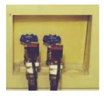
about washing machine hose failure ever again. The *Saf-T-Smart washer valve safety kit* uses a control module that senses water demand, a timer to regulate supply, and two low-voltage solenoids installed directly onto the hot and cold water. One model fits all applications. No plumbing or electrical experience is required.
