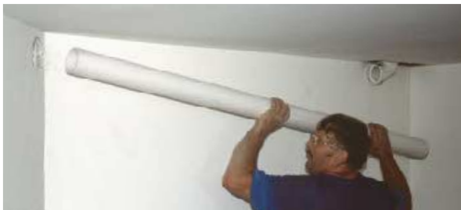
Figure 3. A length of 3-inch PVC — the lower end of which will be cemented into the slab — turns to pass through a partition wall (left). The sanitary tee will accept a second vent pipe leading to the garage. Below, the main vent line continues through a finished portion of the basement (later enclosed in a pipe chase) before exiting through an opening in the band joist. Like plumbing vent pipe, radon venting must be pitched enough to allow condensate and rainwater to drain.
