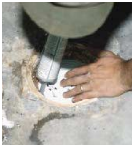
Figure 1. A special check valve is used to prevent the sub-slab ventilation system from sucking indoor air through the floor drain. It opens for drainage when weighted down by accumulated water, but when the drain is dry, a spring-loaded ball provides a seal that maintains negative pressure beneath the slab (left). Once the valve has been cemented in place (center), any visible cracks in the slab or foundation walls are repaired with a durable sealant (right).
