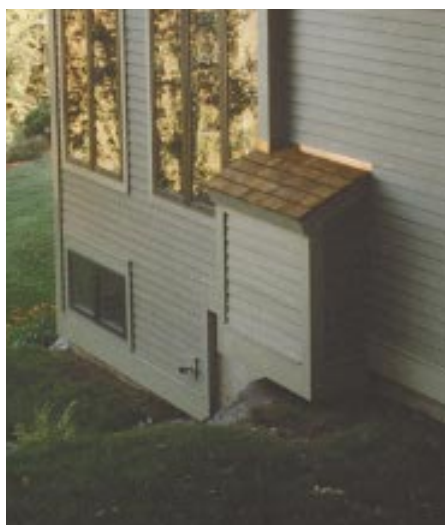
Figure 6. External vents always require a fan to provide a reliable draft. The vent pipe was secured to the fan housing with standard neoprene plumbing connectors before continuing up the wall of the house (left). The finished assembly — located on an inconspicuous outside elevation — was later boxed in for a more finished appearance (right).
