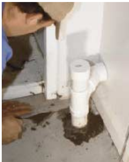
Figure 4. A second hole was hammered into the garage slab to create an additional vent sump (left). The vertical pipe was cemented in place with its open end extending just beneath the underside of the slab, minimizing the risk of blockage by an unexpectedly high water table (right). The uncemented cap on the vent line allows for later expansion, if needed.
