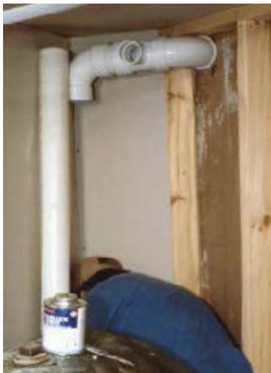
Figure 3. A length of 3-inch PVC — the lower end of which will be cemented into the slab — turns to pass through a partition wall (left). The sanitary tee will accept a second vent pipe leading to the garage. Below, the main vent line continues through a finished portion of the basement (later enclosed in a pipe chase) before exiting through an opening in the band joist. Like plumbing vent pipe, radon venting must be pitched enough to allow condensate and rainwater to drain.
