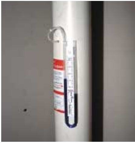
Figure 7. A vacuum monitor installed in the vent pipe confirms that the fan is providing the required negative pressure, although further testing is needed to determine whether indoor radon levels have actually declined.
