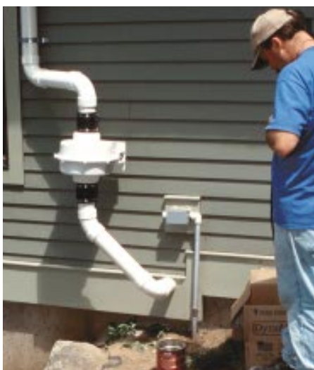
Figure 6. External vents always require a fan to provide a reliable draft. The vent pipe was secured to the fan housing with standard neoprene plumbing connectors before continuing up the wall of the house (left). The finished assembly — located on an inconspicuous outside elevation — was later boxed in for a more finished appearance (right).
