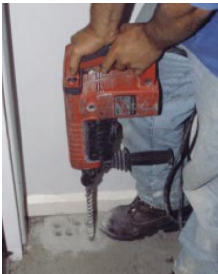
Figure 4. A second hole was hammered into the garage slab to create an additional vent sump (left). The vertical pipe was cemented in place with its open end extending just beneath the underside of the slab, minimizing the risk of blockage by an unexpectedly high water table (right). The uncemented cap on the vent line allows for later expansion, if needed.
