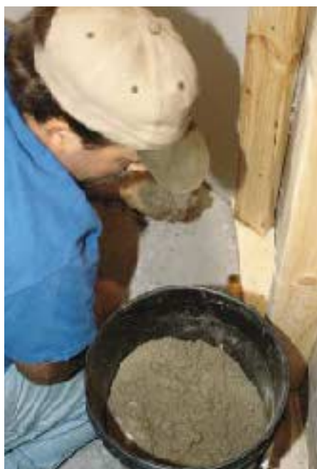
Figure 2. Once a vent opening through the slab has been made with a rotary hammer (left), the fill beneath is dug out to create a sump (center). The finished sump is about a foot deep and as wide as a worker can reach by hand (right).
