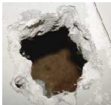
Figure 2. Once a vent opening through the slab has been made with a rotary hammer (left), the fill beneath is dug out to create a sump (center). The finished sump is about a foot deep and as wide as a worker can reach by hand (right).
