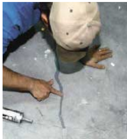
Figure 1. A special check valve is used to prevent the sub-slab ventilation system from sucking indoor air through the floor drain. It opens for drainage when weighted down by accumulated water, but when the drain is dry, a spring-loaded ball provides a seal that maintains negative pressure beneath the slab (left). Once the valve has been cemented in place (center), any visible cracks in the slab or foundation walls are repaired with a durable sealant (right).
