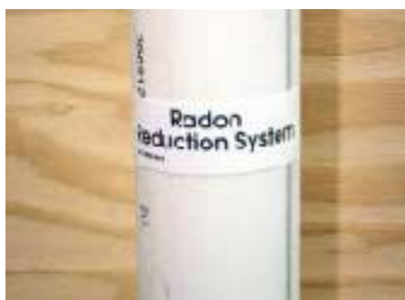
Figure 5. The radon-reduction piping is clearly marked at regular intervals to ensure that it won't be confused with plumbing drains.
