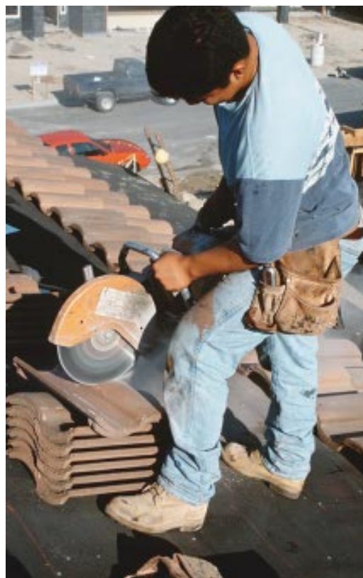
Figure 6. A small corner of tile can often be knocked off with a hatchet (above). Larger cuts are made with a saw equipped with a diamond blade (right).
