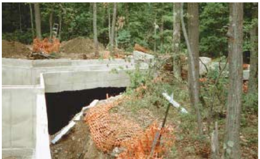
Figure 3. Don't try to save trees that can't be saved. The oaks at the edge of this foundation have lost too many of their roots to survive for more than a few years. It would have been cheaper and much less troublesome to remove them before starting to build.
