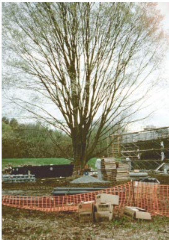
Figure 5. Although the root zone of this tree was defined with snow fencing, lack of adequate site supervision made that a wasted effort (top). The broken limb and damaged bark on the tree at bottom are the most visible injuries, but the excavated material piled beneath it will soon suffocate the roots.
