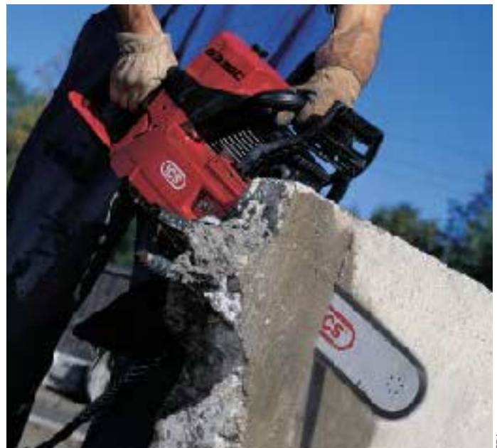
Figure 7. The authors use a gas-powered, plunge-cutting diamond chainsaw for applications where a wall saw is unsuitable, such as completing corner cuts, carving out beam pockets, and sawing through round or irregular concrete.
