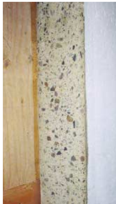
Figure 1. Crisp edges and a smooth, terrazzo-like surface are characteristic of wet-sawn concrete.
