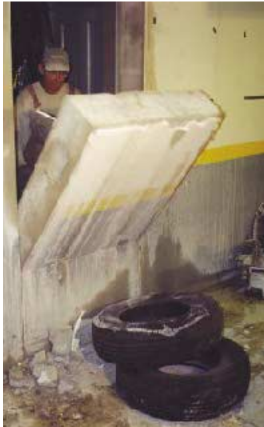
Figure 8. Tires break the impact of a solid-filled CMU wall section to prevent damage to the finished slab.
