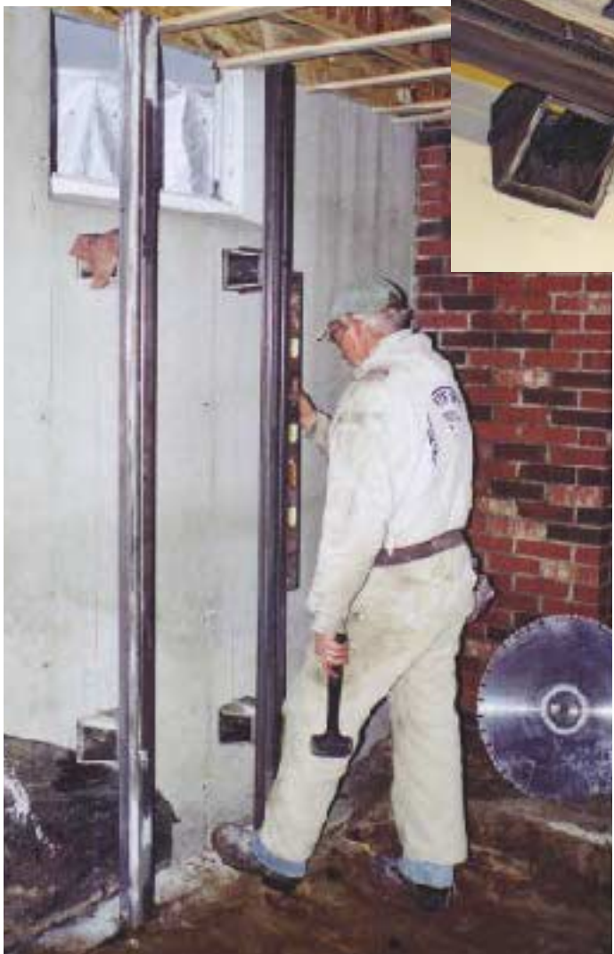
Figure 4. Track mounts are installed and individually leveled for alignment (top). The mounts have a slotted hole that allows the track to be tapped into level after attachment (above). Four adjusting screws in each mount allow the track to be leveled or squared to the cut (inset).
