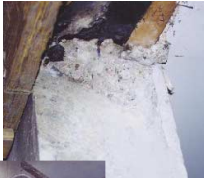
Figure 6. An overhead floor limits a through-cut (above). To avoid a broken "ear" at the top corner, the author scores the backside of the cut with a hand-held cutoff tool (left) and carefully completes the cut with a pneumatic chisel.
