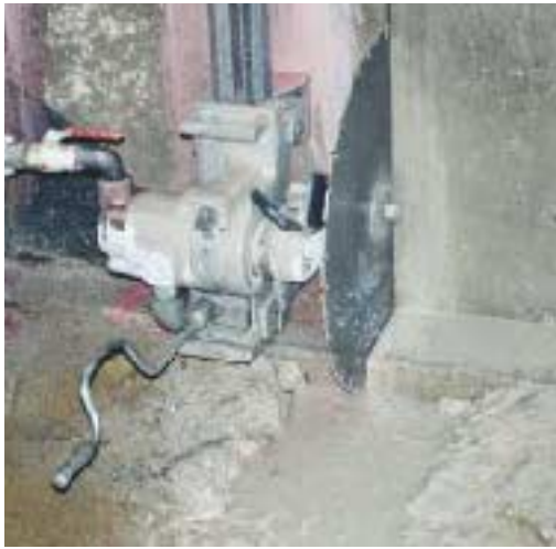
Figure 5. Impeller lube and concrete slurry stain the wall after sawing. The lube (automotive transmission fluid) can be omitted to reduce cleanup when altering a finished interior wall.
