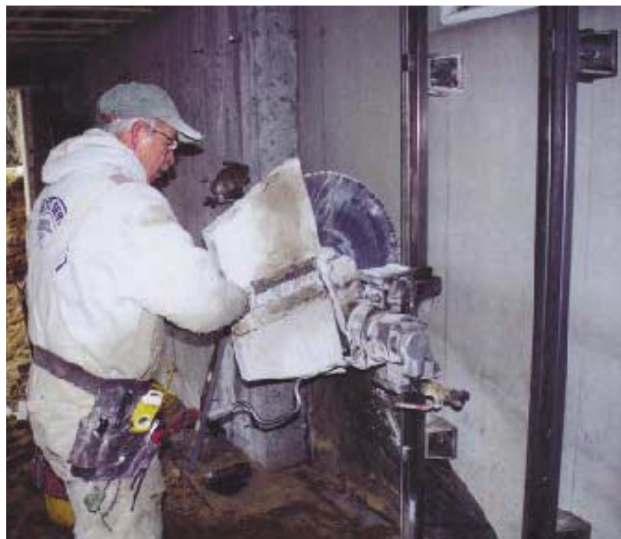
Figure 2. The Cushion Cut diamond wall saw can handle 24- to 42-inch-diameter blades and cuts up to 18 inches deep. It takes about three passes to cut through an 8-inch wall.
