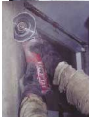
Figure 6. An overhead floor limits a through-cut (above). To avoid a broken "ear" at the top corner, the author scores the backside of the cut with a hand-held cutoff tool (left) and carefully completes the cut with a pneumatic chisel.
