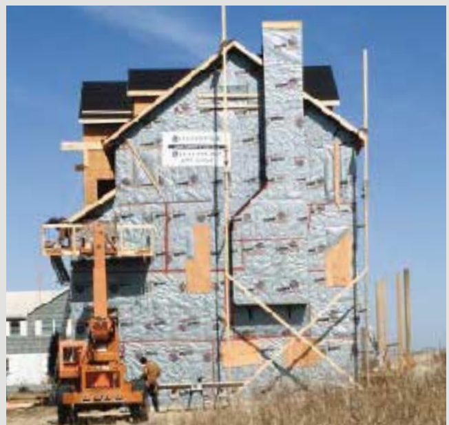
Figure 6. A motorized aerial lift can make quick work out of many overhead jobs. Units rent for $800 to $1,200 a week — possibly less than the cost of the extra manpower required to rig a job manually.
