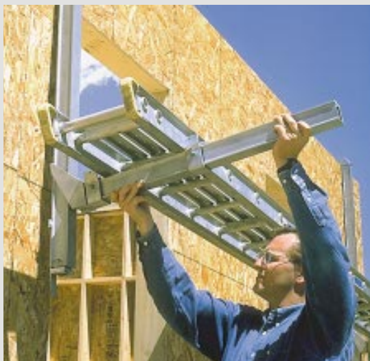
Figure 4. WallWalkers overcome many of the limitations of conventional wall jacks. The unique design can be used on the inside or outside of a wall, and the height can be adjusted without removing staging planks.
