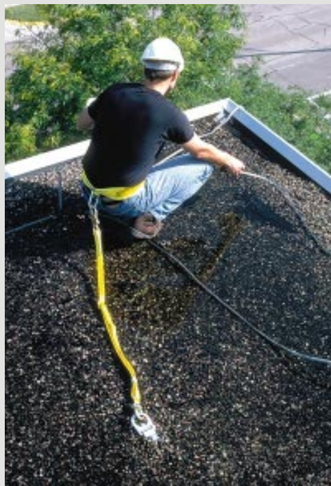
Figure 1. A Personal Fall Arrest System typically consists of an approved building anchor, a body harness, a lifeline, a connecting device, and a lanyard. Many manufacturers bundle the necessary components in a kit like the $163 Compliance in a Can from Protecta Corp. (left). A body belt may be used for restraint or positioning — to prevent a worker from approaching the edge of a flat or low-slope roof, for example — but must never be used where there's a chance that a vertical fall may occur (right).
