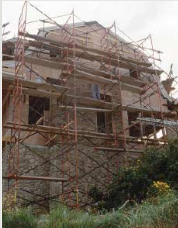
Figure 5. This scaffolding setup looks pretty good, but the planking is an accident waiting to happen. OSHA requires that only approved planking be used (not #2 framing lumber), which must totally fill the space between uprights (1-inch maximum gap). To prevent them from being accidentally dislodged, the individual planks must also be cleated together.
