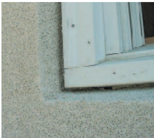
Figure 7. This joint between the EIFS and the brick-mold window casing should be sealed with backer rod and silicone sealant. Apply sealant to the base coat before the finish coat is applied. Be aware that many windows allow water to pass between the casing and the sill or jamb, so that surface joint sealing provides only partial protection. To protect the sheathing and framing, the secondary weather barrier and window flashing must be in place beneath the EIFS and the window.
