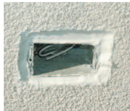
Figure 8. All penetrations should be flashed beneath the EIFS, as well as surface-sealed at the joint. In this example, peel-and-stick membrane is used to seal the electrical box to the housewrap (top left). A gap is left between the EIFS and the box (top middle), and the gap is then filled with backer rod and sealant (top right). Hose bibbs (left) receive a similar treatment.
