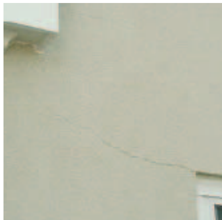
Figure 5. Window corners and narrow intersections between large wall sections are points of stress concentration where cracking may occur. If possible, the design should allow for isolation joints to relieve stress at such locations. In any case, the secondary weather barrier must provide protection for wall materials beneath the EIFS.
