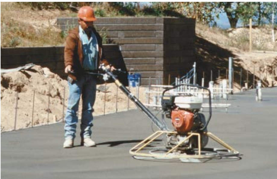
Figure 9. All bleed water should have left the surface before any hand-finishing or power-trowelling begins (above). Even with a power trowel on the job, some hand-finishing is necessary around obstructions (right).
