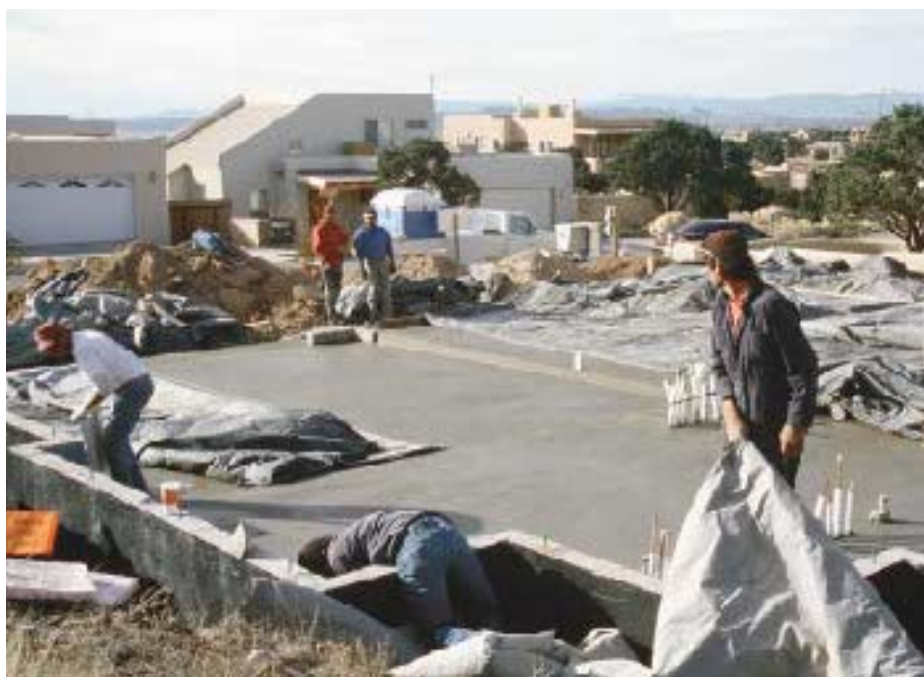
Figure 10. If there is any chance of freezing, blankets are used to protect the subgrade before placing the slab (top), and to cover the fresh concrete for at least three days after (above).
