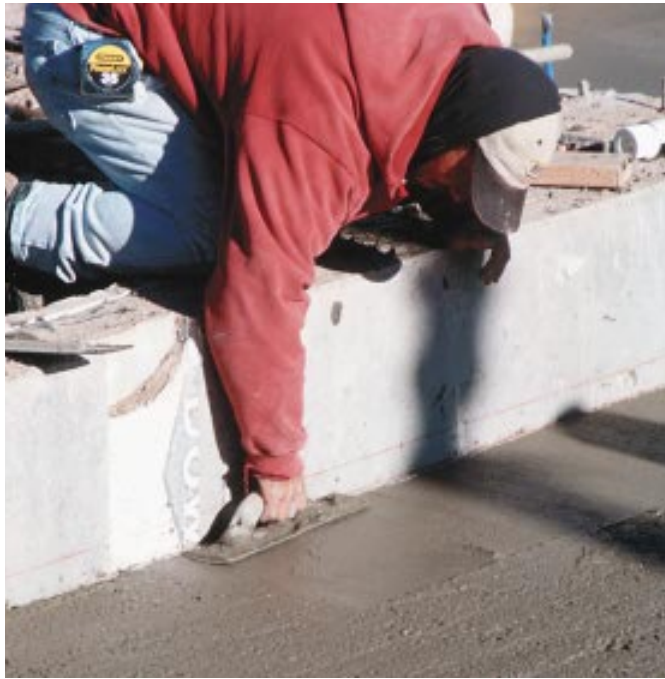
Figure 8. To keep the job moving, it's a good idea to hand-float the slab perimeter as the concrete is placed.
