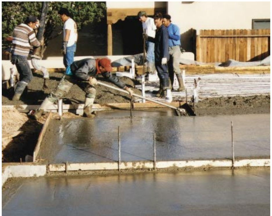
Figure 7. Concrete should be bull-floated as soon as it has been screeded (left). Bleed water will begin to appear soon after (below), but make sure it's gone before finishing begins.
