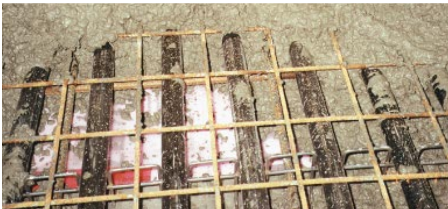
Figure 5. Placing rebar and pipes so concrete can flow underneath them prevents stress risers.
