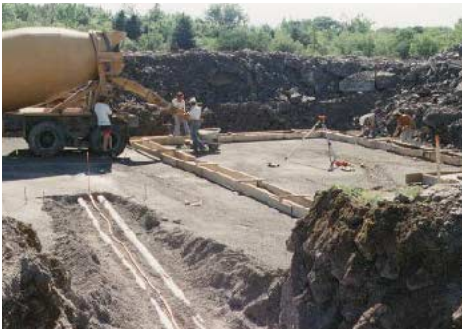
Figure 1. A properly prepared subgrade should be uniformly compacted across the full area of the slab, leveled to within 1/2 inch.
