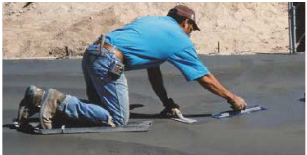
Figure 9. All bleed water should have left the surface before any hand-finishing or power-trowelling begins (above). Even with a power trowel on the job, some hand-finishing is necessary around obstructions (right).
