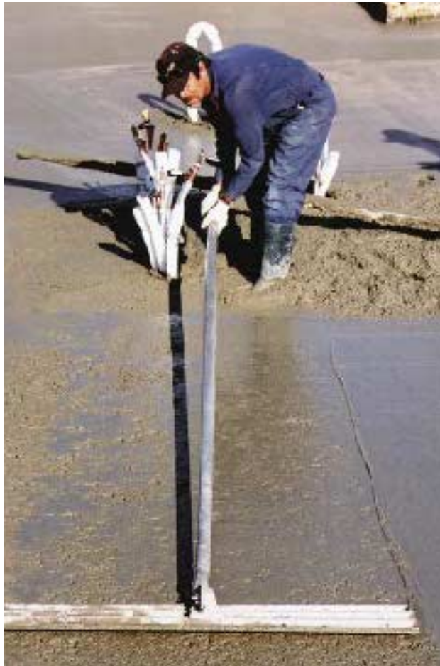
Figure 7. Concrete should be bull-floated as soon as it has been screeded (left). Bleed water will begin to appear soon after (below), but make sure it's gone before finishing begins.
