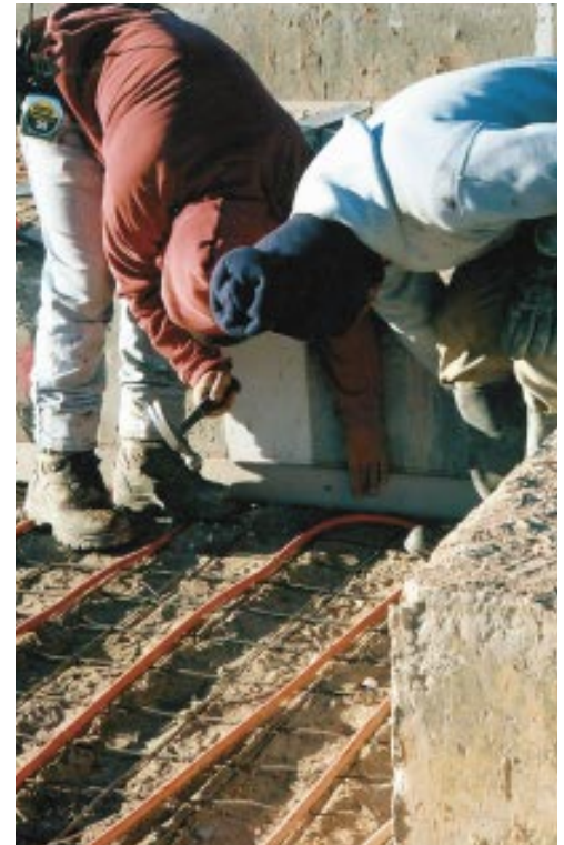
Figure 3. Fiberboard expansion joint material permits the slab to move independently of the wall (photo, right). For a finished appearance at the slab edge, score the fiberboard on a table saw so the top 1/2 inch can be easily snapped off after the pour. Then finish the joint with sealant (above).
