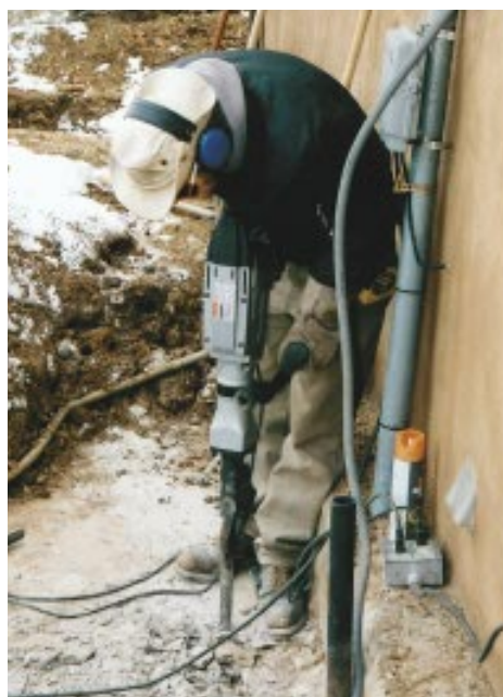
Figure 1. These lighter hammers are ideal for surgical demolition, like locating water lines that are right near the electrical service.
