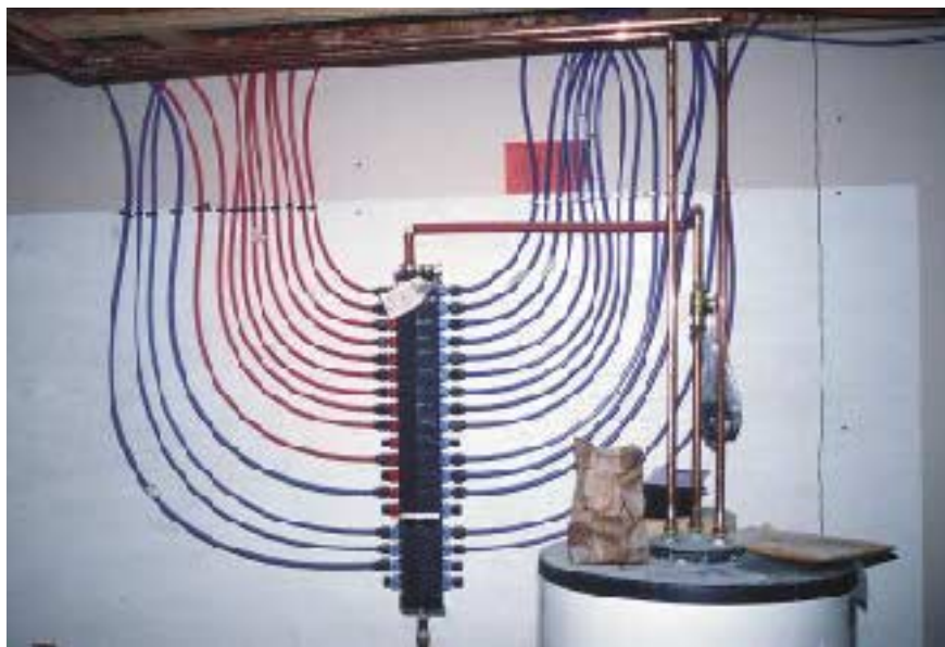
When using PEX to supply domestic water, most manufacturers recommend connecting each fixture using home-run supply pipes that originate at a central manifold.
