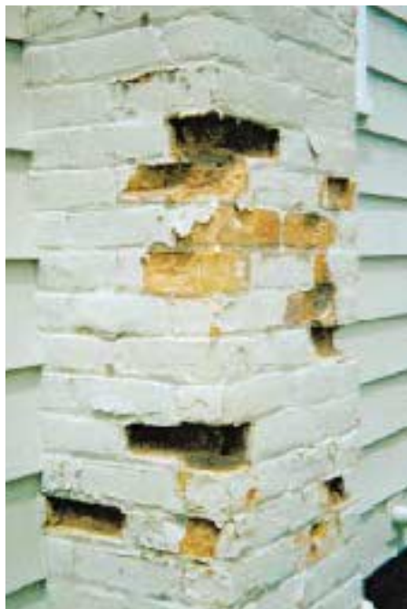
Masonry chimneys can be damaged when corrosive flue gases condense in cold, oversized flues. Exterior chimneys like this one are particularly subject to condensation.
