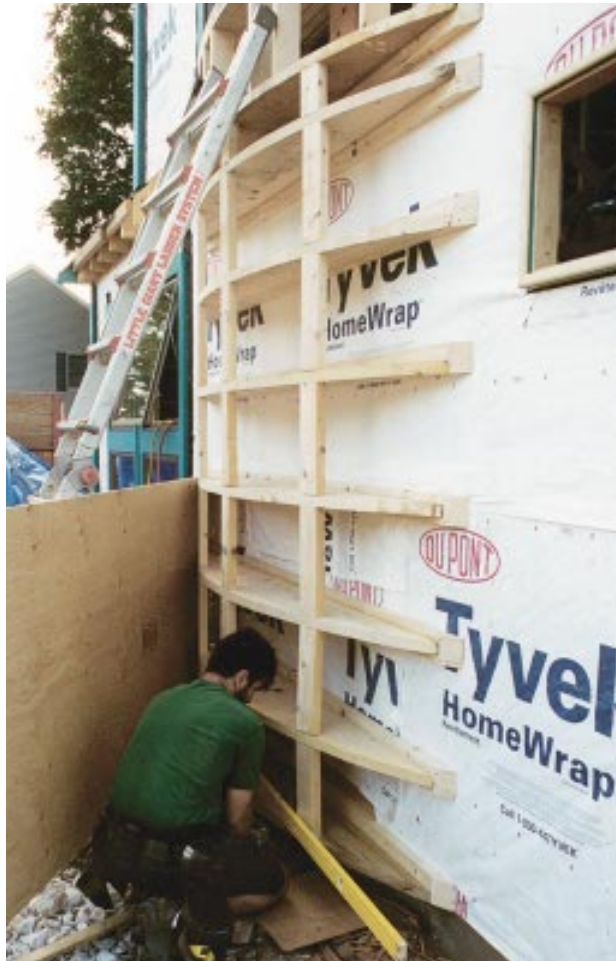
Curved 2x10 nailers, cut on a band saw, define the exterior radius.
