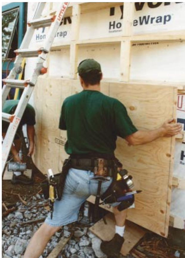
Because the curve is gentle, bending 1/2-inch plywood sheathing was easy.
