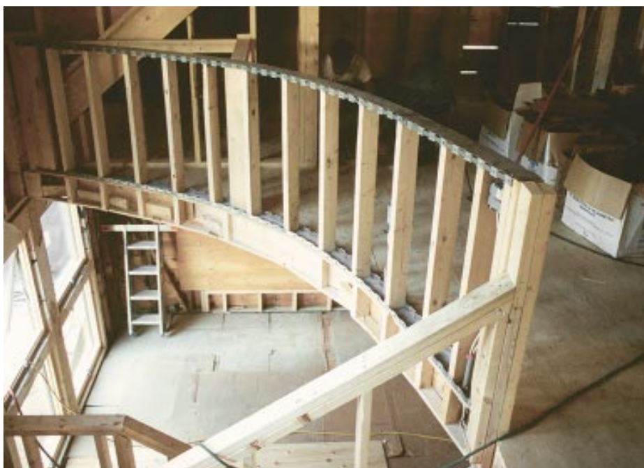
Flex-C Trac metal plates save the time required to lay out and cut plywood plates. Studs attach easily with screws.
