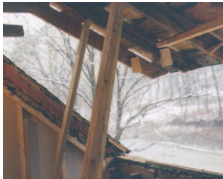
Figure 3. As the roof swings up, the rafter tails swing out, so the jacking point must be repositioned inward.
