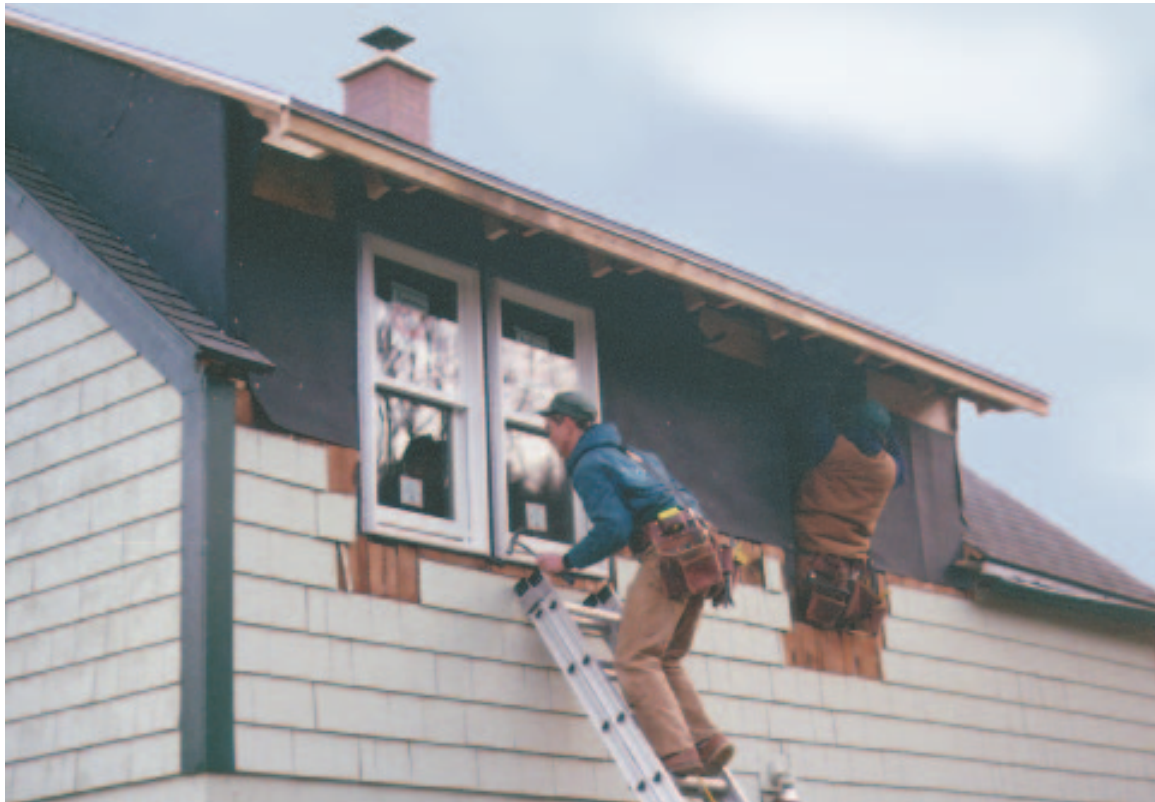
Figure 4. New double-hung windows, sidewall shingles, and chimney top complete the exterior of the dormer.
