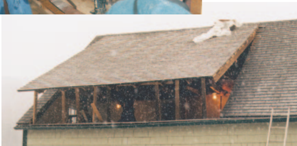
Figure 2. With the rafters cut free of the kneewall plate, hydraulic jacks ease the roof up to its new elevation (left). Even as the roof gapes open, most of the weather is kept outside.
