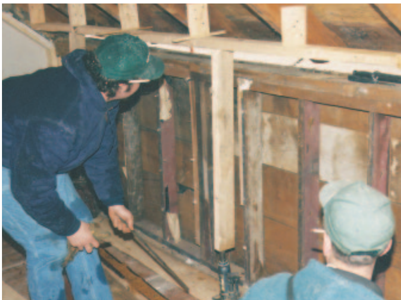
Figure 2. With the rafters cut free of the kneewall plate, hydraulic jacks ease the roof up to its new elevation (left). Even as the roof gapes open, most of the weather is kept outside.
