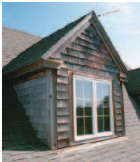
Figure 2. To look proportionate, trim details should be downsized on doghouse dormers. A 25% reduction looked right in this case.
