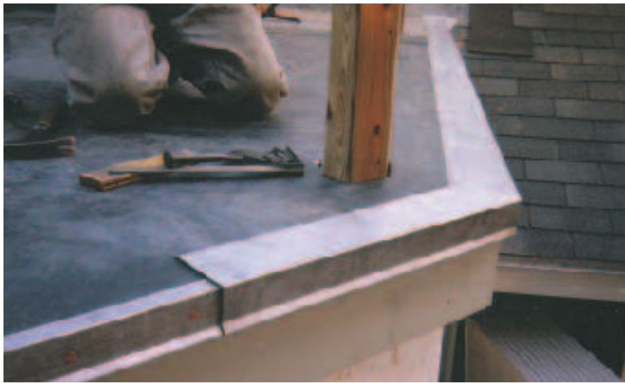
Figure 4. A custom-made two-piece lead-coated copper drip-edge conceals face-driven fasteners. The drip-edge will be sealed to the membrane with a 6-inch-wide rubber cover strip.
