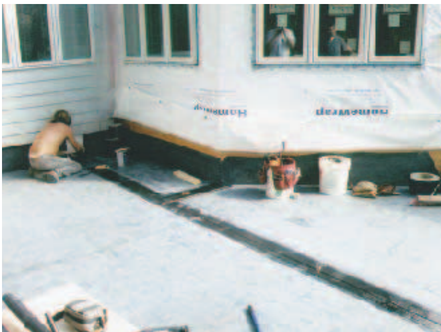
Figure 3. The overlapping seams in an EPDM membrane are treated separately from the main bonding operation. After brushing the seam with primer, the author applies a pressure-sensitive seam tape to secure and seal the edge (top). As a redundant fail-safe measure, the author applies a 6-inch-wide peel-and-stick rubber flashing strip over every seam in the membrane and seals the strip's edges with a lap sealant (above).
