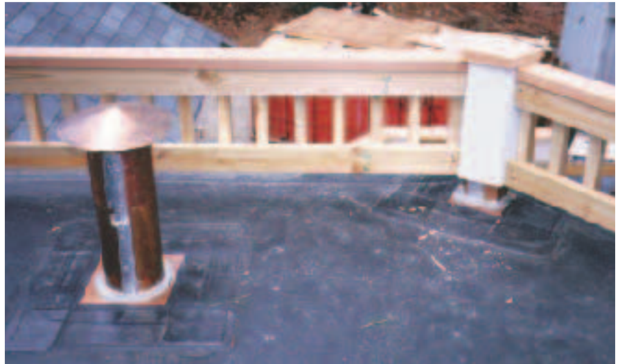
Figure 6. The roofing contractor installed custom flanged copper sleeves over the railing posts and plumbing vent. The flange is bedded in sealant on top of the EPDM membrane, then tightly covered under peel-and-stick rubber flashing strips.
