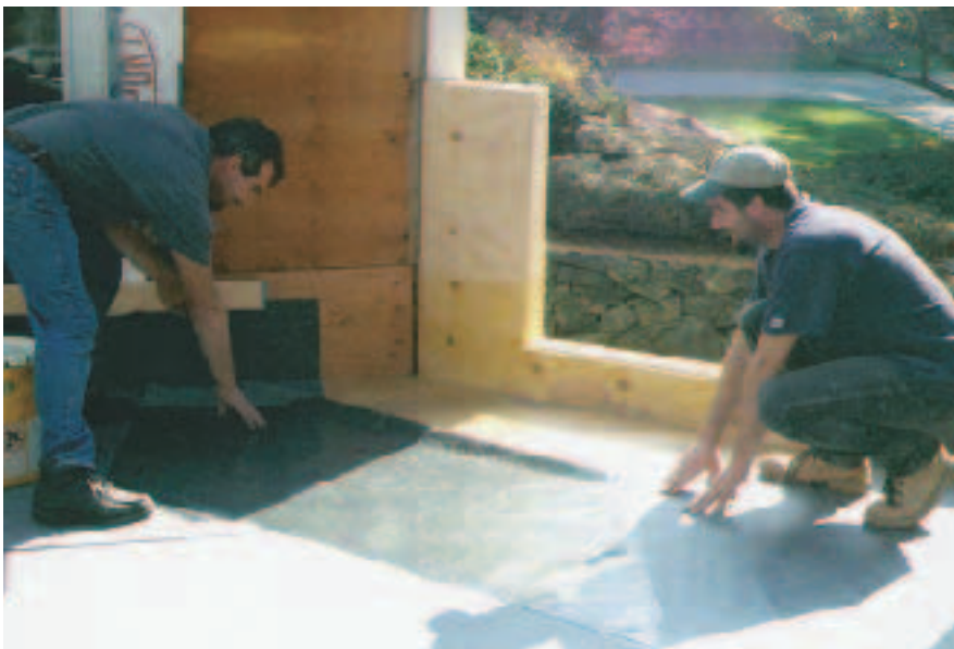
Figure 1. Four hands are better than two to prevent wrinkles and trapped air bubbles in the EPDM bonding process.
