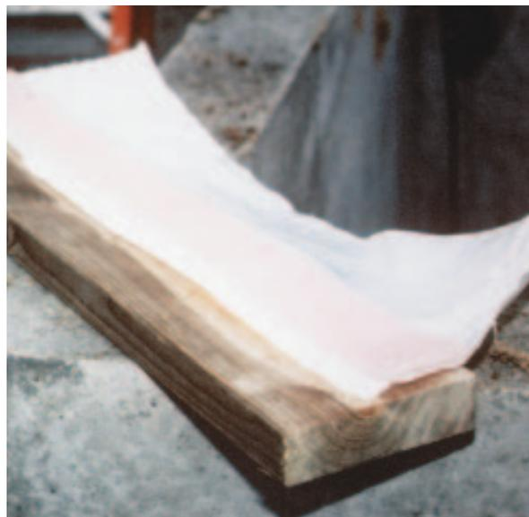
**Figure 4.** Before installing the mudsill, a 6-inch-wide strip of poly is embedded in Tremco sealant and stapled to the underside. A 2¾-inch-wide strip of foam sill seal is stapled over the poly, and then the sill is flipped over and bolted in place. The poly flap faces the exterior.
