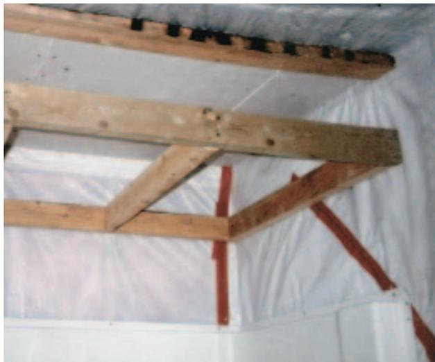
**Figure 13.** When planning for a light fixture above a tub, it sometimes makes sense to lower the ceiling to keep the electrical box from penetrating the poly ceiling barrier.
