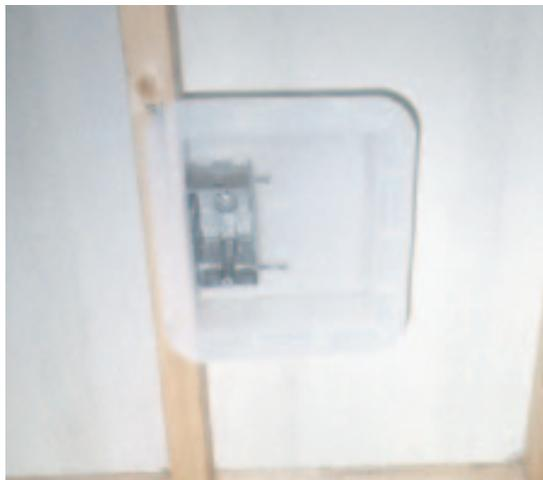
**Figure 9.** The Lessco box is a  $6\frac{1}{2} \times 7\frac{1}{2} \times 2\frac{7}{8}$ -inch airtight plastic box that's installed at the same time as a regular electrical box (left). After a wall is insulated, the poly air barrier is taped to the flange of the Lessco box (below), and the Lessco box is insulated with scraps of fiberglass or cellulose. Note that all plumbing penetrations in the wall are sealed with contractor's tape.
