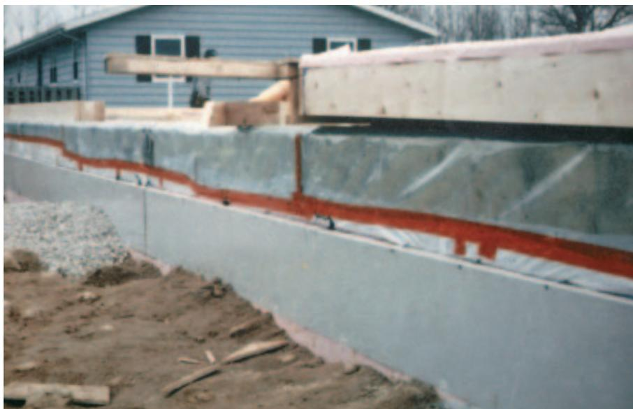
**Figure 5.** The band joist is wrapped with Tenoarm, a very tough, transparent polyethylene. The Tenoarm has been taped to the white polyethylene stapled to the bottom of the mudsill, and then wrapped up onto the subfloor.
