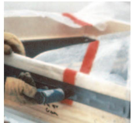
**Figure 14.** A polyethylene “bib” is added around the exterior of each window before it’s installed. Several extra pleats of poly are provided at the window corners (left), so that it can later be folded flat against the interior of the studs. A strip of duct tape over the poly (right) provides reinforcement for the staple heads.
