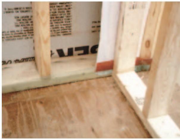
**Figure 11.** In homes where the ceiling poly can't be installed in a single sheet, it's installed room by room. When building the top-floor partitions, the framers must install a strip of poly between the top plates and the ceiling joists. Later, the ceiling poly in each room will be taped to the perimeter flaps.
