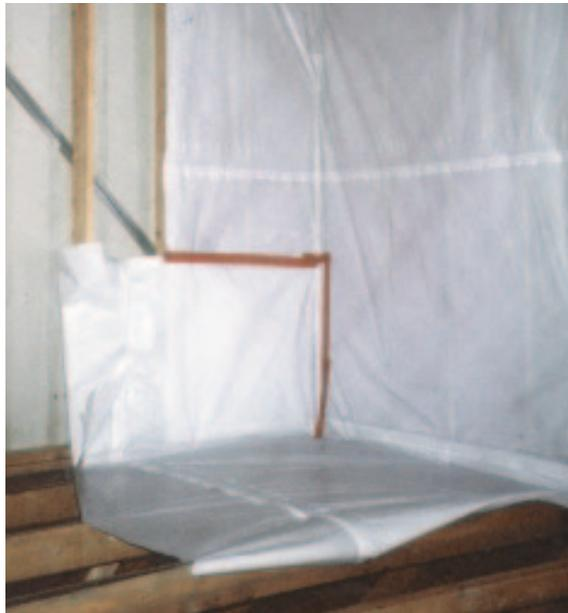
**Figure 8.** If a tub-shower unit is located against an exterior wall, fiberglass insulation and the poly air barrier need to be installed before the tub. All seams in the poly air barrier are taped with red contractor's tape from 3M.
