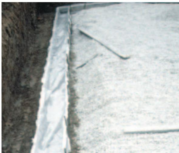
**Figure 2.** In preparation for pouring the basement slab, a layer of 1-inch-thick polystyrene insulation is installed over 6-mil polyethylene and 8 inches of crushed stone.
