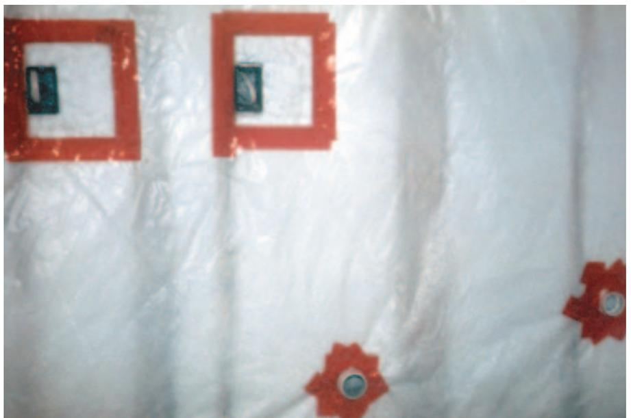
**Figure 10.** Where a partition intersects an exterior wall, a strip of poly is installed on top of the 2x8 drywall nailer before the partition is built. Note that the wall poly is taped to the Tenoarm poly that protrudes from under the bottom plate.
