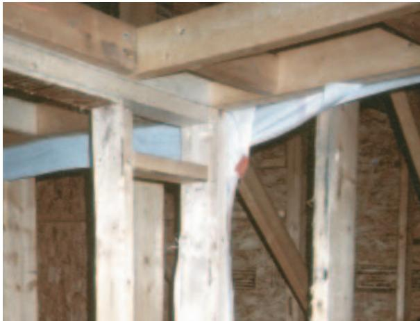
**Figure 12.** A conventional recessed can fixture can be installed in a site-built foam box. The box, which is sized to provide 2 inches of free air on all sides of the fixture, is assembled with Tremco to seal the seams.
