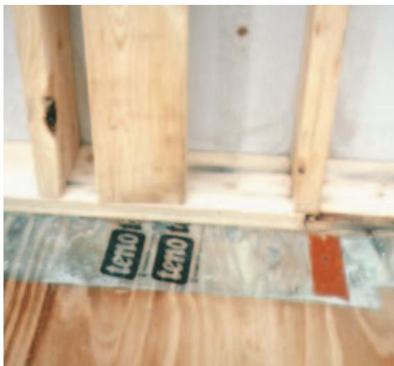
**Figure 7.** To keep the air from the soffit vents from disturbing the attic insulation, flaps of poly are stapled between the heels of the attic trusses. The vent channel only needs to extend above the expected depth of attic insulation.
