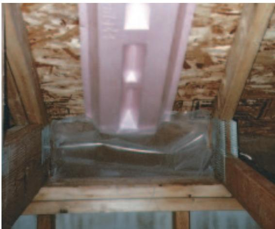
perimeter, I install several layers of rigid foam insulation between the rafters above the wall plates.
