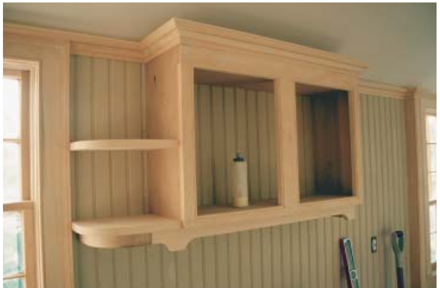
Figure 4. Wall cabinet sides run long to support an undercabinet light valance, which returns around curved open shelving to the wall.
