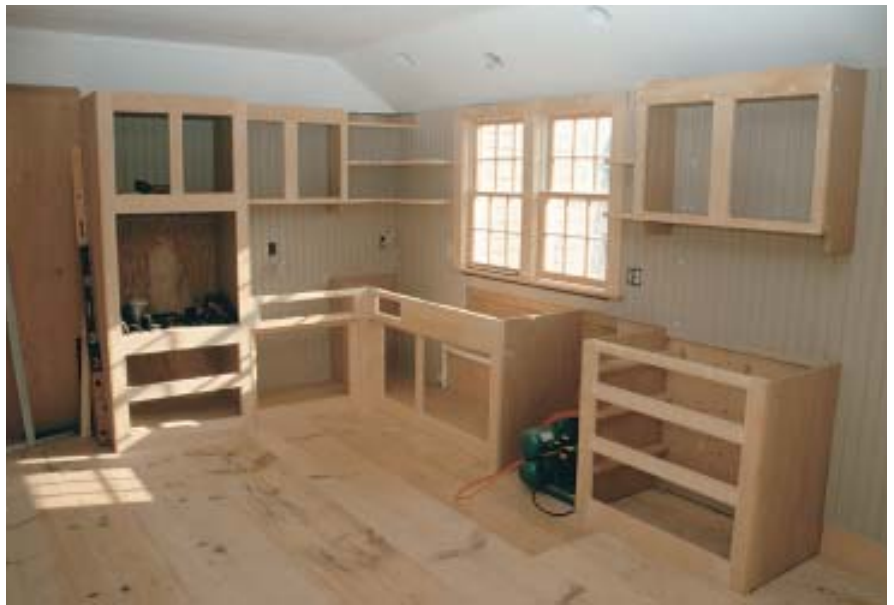
Figure 1. To match the budget, the author used clear, 5/4 sugar pine for the face frames on this job, although he prefers maple for its hardness, stability, and paintability.
