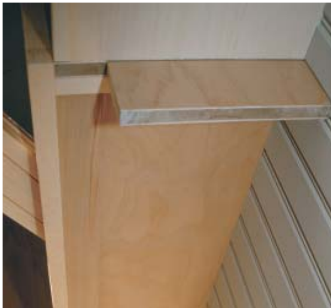
Figure 3. The author installs the beaded paneling after fitting the cabinets to the wall, letting the beaded profile die neatly into the carcass. The wall cabinet sides drop beyond the bottom by 2 inches, forming stops for an undercabinet lighting valance.
