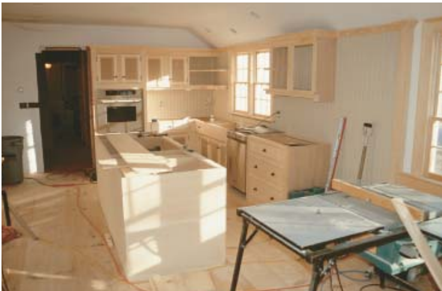
Figure 7. The author prefers to install all finish hardware prior to painting, to determine the best appearance and eliminate the need to patch holes in the finish.
