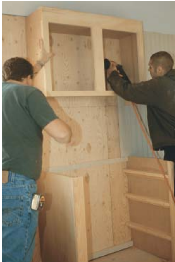
Figure 2. AC plywood replaces the drywall behind the cabinets to provide uninterrupted fastening for the cabinets and beaded wall paneling.
