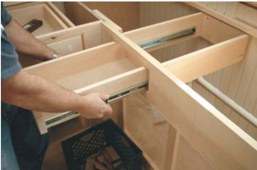
Figure 6. A support frame simplifies hardware installation and drawer alignment. The author premounts the slides on drawer and frame, then aligns and screws the sub-assembly into place before the countertops are installed.
