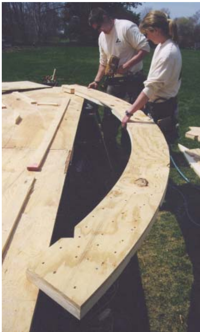
Figure 3. The first layer of plywood was glued and tacked to the 2x12 core, which was then moved to the edge of the work platform and fastened according to the engineer's specifications (above). The assembly was turned over and the protruding nails clinched (top right), then the second layer of plywood was fastened in place with more construction adhesive and three additional rows of nails, offset from those driven from the other side (bottom right).
