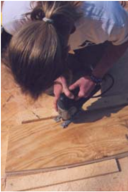
Figure 4. The rafter tails were cut with a circular saw, but seat cuts were made with a jigsaw to prevent overcutting (left). Starter holes in the platform simplified the cuts, and aligning each rafter with the layout lines ensured accuracy (right).
