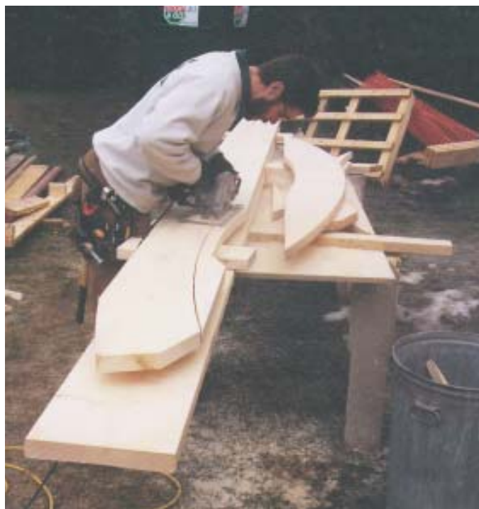
Figure 1. The crew first tried cutting the curved rafters by hand with a circular saw. The technique was fairly accurate but slow.
