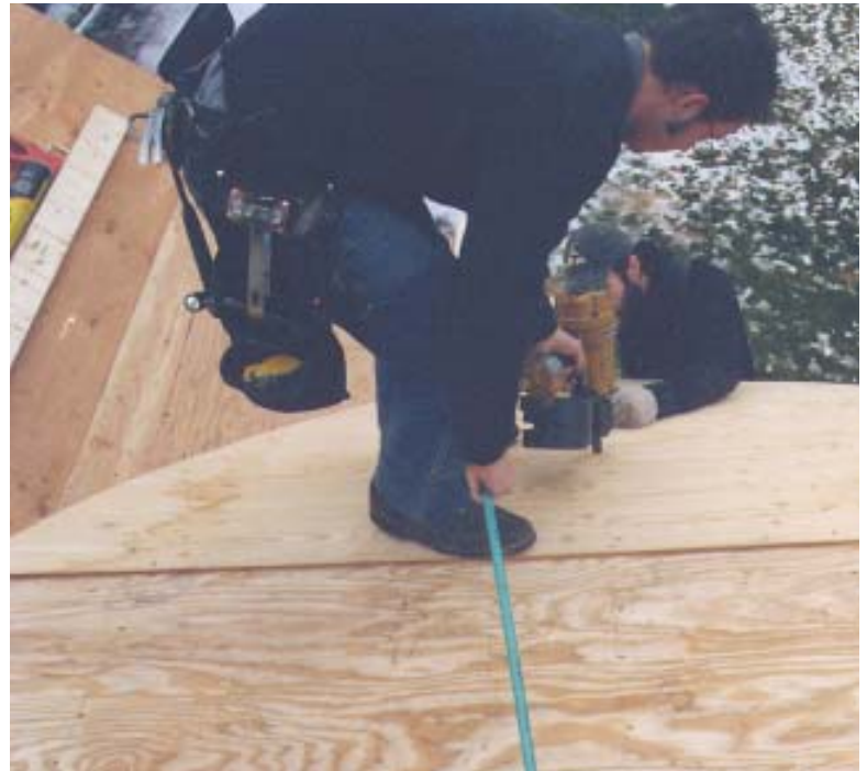
Figure 5. The birdsmouth cuts in the main rafters sat on short girders, while a deeper pair of subrafters was nailed in below to create an arched soffit at the front of the entryway (left). The completed roof frame was sheathed with two layers of \frac{3}{8} -inch plywood (above).
