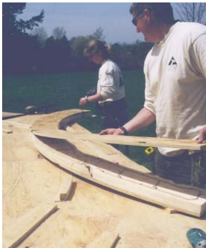
Figure 3. The first layer of plywood was glued and tacked to the 2x12 core, which was then moved to the edge of the work platform and fastened according to the engineer's specifications (above). The assembly was turned over and the protruding nails clinched (top right), then the second layer of plywood was fastened in place with more construction adhesive and three additional rows of nails, offset from those driven from the other side (bottom right).
