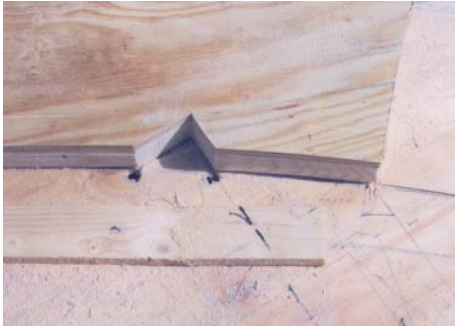
Figure 4. The rafter tails were cut with a circular saw, but seat cuts were made with a jigsaw to prevent overcutting (left). Starter holes in the platform simplified the cuts, and aligning each rafter with the layout lines ensured accuracy (right).
