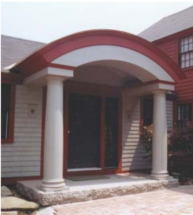
Figure 6. The completed portico was finished with curved trim that was laid out and cut on the same work platform used for building the rafters.
