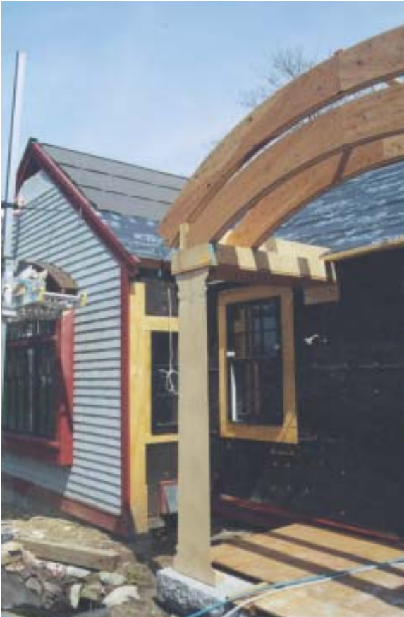
Figure 5. The birdsmouth cuts in the main rafters sat on short girders, while a deeper pair of subrafters was nailed in below to create an arched soffit at the front of the entryway (left). The completed roof frame was sheathed with two layers of \frac{3}{8} -inch plywood (above).
