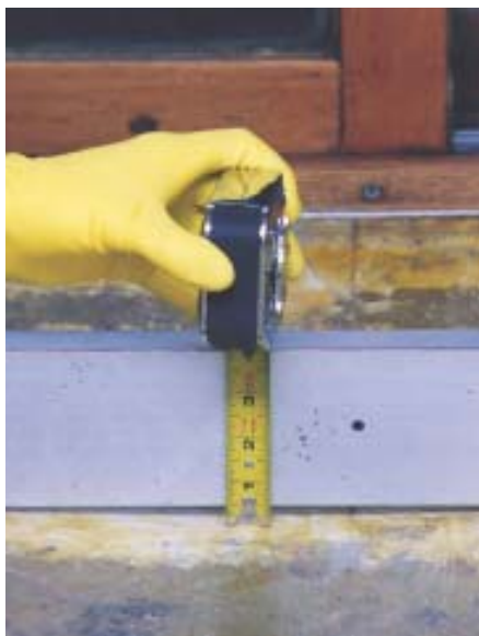
Figure 1. Laminate flooring can be applied over a variety of substrates, including existing flooring materials, as long as the surface is flat enough. Surface irregularities that exceed \frac{3}{16} inch in a 6-foot span must be filled or cut down. Acrylic- or latex-fortified cement-based floor patching material used to fill low spots should be tapered to a feather edge.
