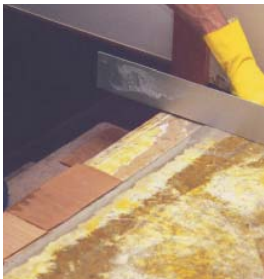
Figure 2. Minor low spots can be corrected with several layers of 15-pound felt (above). Cutting each successive piece smaller than the one before builds up the greatest thickness in the center and tapers the edges. If necessary, the felt can be taped in place until the weight of the laminate floor holds it in place permanently. The author also uses cedar shims to ease transitions at doors and stairways (right).
