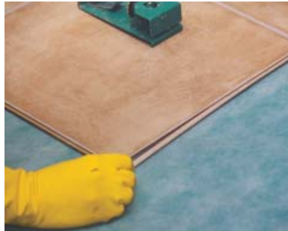
Figure 7. Tiles are typically installed from left to right, beginning with a grooved side against the wall. Slip tongues are used to change direction where needed to avoid an inefficient "backfill" installation.
