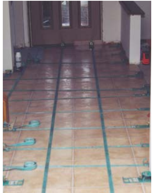
Figure 6. Proprietary strap clamps secure the first rows of flooring (above). Clamps can be adjusted to alter the spacing between the edge of the flooring and the adjacent wall to compensate for any irregularities in the framing. A carefully aligned initial strip of flooring several tiles wide is glued, clamped, and allowed to set up for an hour. Clamps are then loosened and retightened as needed to place additional tiles (right).
