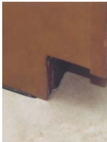
Figure 9. To eliminate the need for quarter-round at the base of the toe kick, the author scribes the combined thickness of the flooring and underlayment on the outside corners (left), which are then slightly undercut (center) and cleaned out with a chisel. Leaving a small amount of extra material in the corner of the adjoining L-shaped tile lets the flooring dive under the corner for a clean look with no visible gap (right). The expansion gap in the kickspace is covered with vinyl cove base, which is cut off flush with the side of the cabinet. The gap at the side is concealed by quarter-round that terminates just short of the corner with a back cut.
