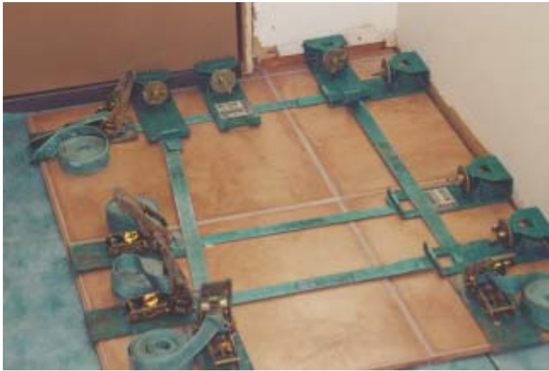
Figure 6. Proprietary strap clamps secure the first rows of flooring (above). Clamps can be adjusted to alter the spacing between the edge of the flooring and the adjacent wall to compensate for any irregularities in the framing. A carefully aligned initial strip of flooring several tiles wide is glued, clamped, and allowed to set up for an hour. Clamps are then loosened and retightened as needed to place additional tiles (right).
