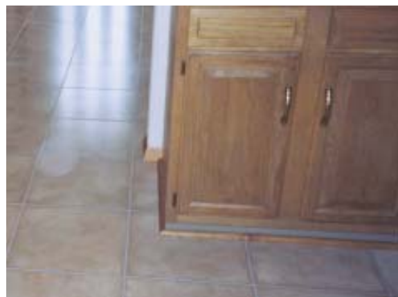
Figure 8. Quarter-round trim strips are fastened to cabinet bases to conceal the required 1/4-inch expansion gap between flooring and base. The kickspace can be finished with vinyl cove base.
