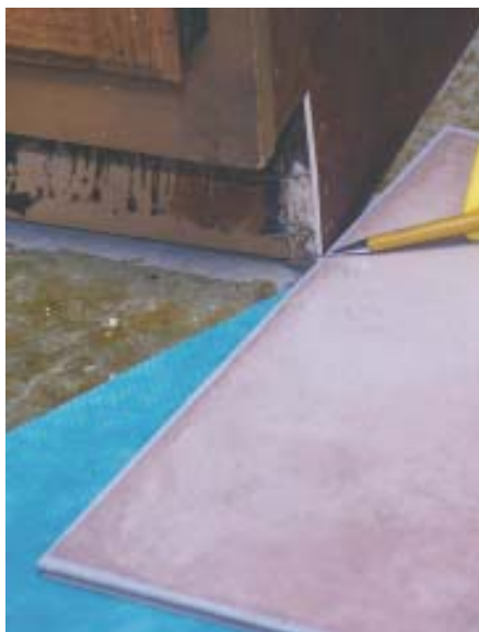
Figure 9. To eliminate the need for quarter-round at the base of the toe kick, the author scribes the combined thickness of the flooring and underlayment on the outside corners (left), which are then slightly undercut (center) and cleaned out with a chisel. Leaving a small amount of extra material in the corner of the adjoining L-shaped tile lets the flooring dive under the corner for a clean look with no visible gap (right). The expansion gap in the kickspace is covered with vinyl cove base, which is cut off flush with the side of the cabinet. The gap at the side is concealed by quarter-round that terminates just short of the corner with a back cut.
