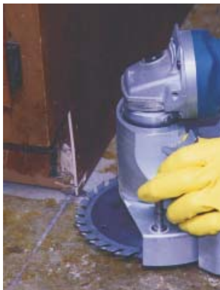
Figure 9. To eliminate the need for quarter-round at the base of the toe kick, the author scribes the combined thickness of the flooring and underlayment on the outside corners (left), which are then slightly undercut (center) and cleaned out with a chisel. Leaving a small amount of extra material in the corner of the adjoining L-shaped tile lets the flooring dive under the corner for a clean look with no visible gap (right). The expansion gap in the kickspace is covered with vinyl cove base, which is cut off flush with the side of the cabinet. The gap at the side is concealed by quarter-round that terminates just short of the corner with a back cut.
