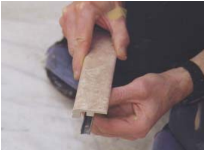
Figure 11. Transitions between laminate flooring and carpeting require a two-piece carpet reducer (top left). After the U-shaped metal base is fastened to the concrete subfloor with expansion anchors and screws (top right), the transition piece itself snaps into place. In a neat-looking installation, the lip of the trim piece should be pressed snugly against the carpet (right). If the height difference is too great — which is often the case where thin, dense carpeting is used — it may require “ramping up” the edge of the carpet to the proper height with cedar-shingle shims between carpet pad and subfloor.
