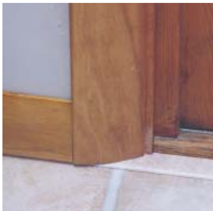
Figure 10. Here, the author trims the transition between flooring and a sliding door threshold with end molding (above). The vertical leg of the trim piece is embedded in a bead of silicone caulk in the gap between flooring and threshold; undercutting the side casings makes it possible to slip the molding beneath them, eliminating the need for complicated scribe cuts. End molding can also be used to trim the base of a carpeted riser (above right). If the gap between flooring and riser is sized correctly, the pressure from the carpeted riser will hold the trim piece firmly in place but still allow the floor to move (right).
