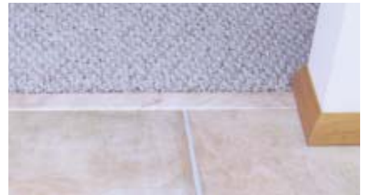
Figure 11. Transitions between laminate flooring and carpeting require a two-piece carpet reducer (top left). After the U-shaped metal base is fastened to the concrete subfloor with expansion anchors and screws (top right), the transition piece itself snaps into place. In a neat-looking installation, the lip of the trim piece should be pressed snugly against the carpet (right). If the height difference is too great — which is often the case where thin, dense carpeting is used — it may require “ramping up” the edge of the carpet to the proper height with cedar-shingle shims between carpet pad and subfloor.
