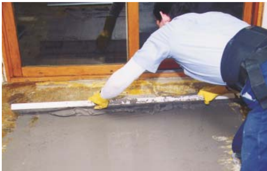
Figure 1. Laminate flooring can be applied over a variety of substrates, including existing flooring materials, as long as the surface is flat enough. Surface irregularities that exceed \frac{3}{16} inch in a 6-foot span must be filled or cut down. Acrylic- or latex-fortified cement-based floor patching material used to fill low spots should be tapered to a feather edge.
