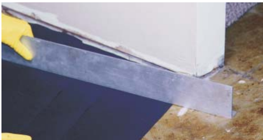
Figure 2. Minor low spots can be corrected with several layers of 15-pound felt (above). Cutting each successive piece smaller than the one before builds up the greatest thickness in the center and tapers the edges. If necessary, the felt can be taped in place until the weight of the laminate floor holds it in place permanently. The author also uses cedar shims to ease transitions at doors and stairways (right).
