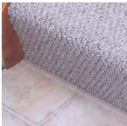
Figure 10. Here, the author trims the transition between flooring and a sliding door threshold with end molding (above). The vertical leg of the trim piece is embedded in a bead of silicone caulk in the gap between flooring and threshold; undercutting the side casings makes it possible to slip the molding beneath them, eliminating the need for complicated scribe cuts. End molding can also be used to trim the base of a carpeted riser (above right). If the gap between flooring and riser is sized correctly, the pressure from the carpeted riser will hold the trim piece firmly in place but still allow the floor to move (right).
