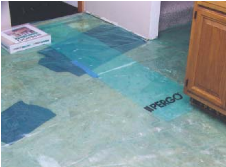
Figure 3. All laminate flooring manufacturers require a poly vapor barrier if the laminate will be applied over a concrete subfloor. Adjoining sheets of poly should be taped in position and must overlap by at least 8 inches (left). The vapor barrier is followed by a foam underlayment that provides cushioning and compensates for any remaining irregularities in the subfloor. Pergo offers the choice of a standard-grade underlayment (on top in the bottom photo) or a denser premium-grade material (underneath).
