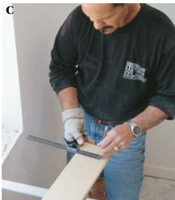
Figure 8. With the stool supported by aluminum window sticks, the blade of a combination square is aligned with the window return to transfer the required cut to the stool (A). The depth of the notch cut is then picked up with the square (B) and scribed onto the stool (C) before the notch is cut out with a cordless jigsaw.
