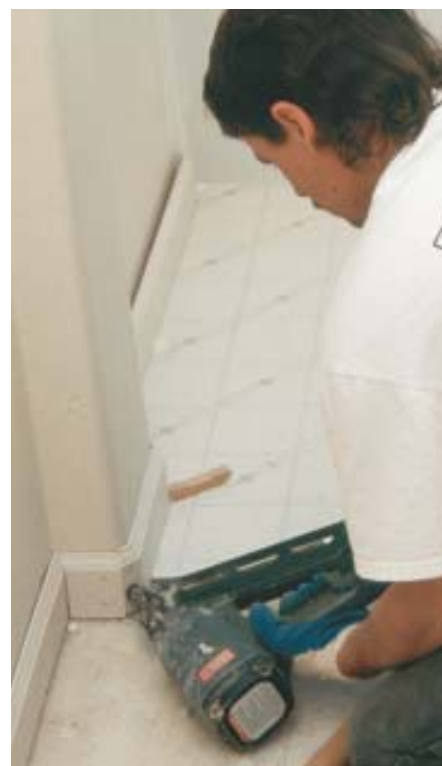
Figure 7. The small filler pieces needed to wrap bull-nosed corners are tough to nail safely, so they're temporarily held in place with hot-melt glue.
