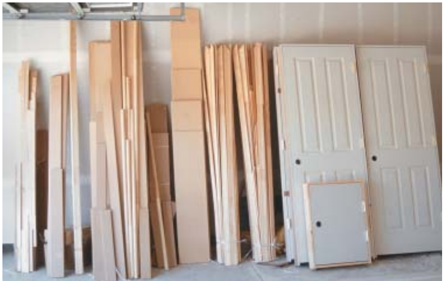
Figure 2. The partially prepared trim package is delivered to each house, where the first task of the trim carpenters is to break it down and distribute the material from room to room.
