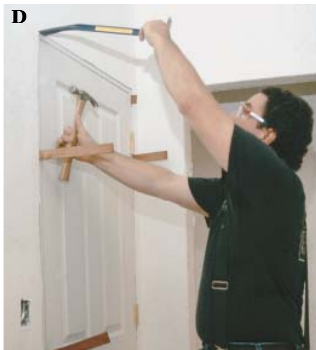
Figure 4. The first step in installing an interior door is to shoot a couple of nails into the top of the hinge side of the jamb. Leaving space between the jamb and the framing at this stage makes it easy to drive shims into place later (A). After the shims are in place, the door should open and close freely without hitting the jamb or binding at the hinge (B). Adjustments are simple to make if the jamb is allowed to float until everything lines up correctly. A soft rubber mallet helps to bring the jamb into alignment with the opening without marring or denting the material (C). The head-jamb reveal is easily adjusted with a flat bar after the jamb is tacked in position (D).
