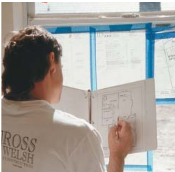
Figure 1. Builder option lists show all products and details that deviate from the standard spec. Good builders post them in the home to spell out the options that the homeowner has chosen, allowing the author's crew to confirm that the correct materials package has been delivered.
