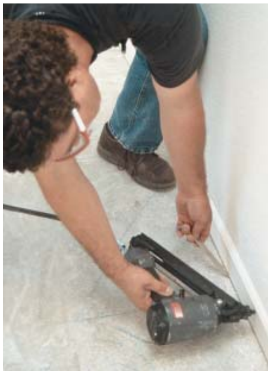
Figure 6. In areas that will be carpeted later, the base is held \frac{3}{8} inch above the floor with a mini pry bar as it's tacked in place.
