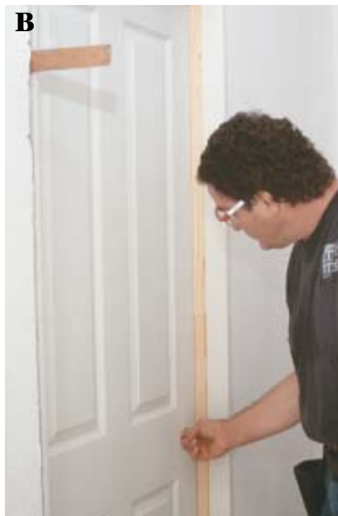
Figure 4. The first step in installing an interior door is to shoot a couple of nails into the top of the hinge side of the jamb. Leaving space between the jamb and the framing at this stage makes it easy to drive shims into place later (A). After the shims are in place, the door should open and close freely without hitting the jamb or binding at the hinge (B). Adjustments are simple to make if the jamb is allowed to float until everything lines up correctly. A soft rubber mallet helps to bring the jamb into alignment with the opening without marring or denting the material (C). The head-jamb reveal is easily adjusted with a flat bar after the jamb is tacked in position (D).
