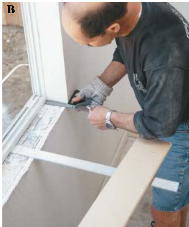
Figure 8. With the stool supported by aluminum window sticks, the blade of a combination square is aligned with the window return to transfer the required cut to the stool (A). The depth of the notch cut is then picked up with the square (B) and scribed onto the stool (C) before the notch is cut out with a cordless jigsaw.
