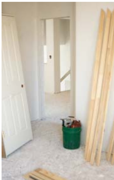
Figure 3. The author's tool bucket and the materials to install and trim a door are perfectly placed to reduce needless effort. One carpenter will install the door, and another will follow to install the trim package.
