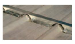
roof, that method tends to fail catastrophically in storms because purlins and hat sections rest on the ribs of the underlying roof. The ribs deflect under high winds, and the fasteners are quickly loosened. Roof Huggers are made to work with the most
