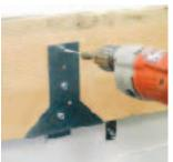
required in most applications, and the labor-intensive marking and drilling of the ledger are eliminated. The connectors for steel framing list for \$8.40 each, and the wood and LVL series list for \$16.80 each. Fasteners are included with the hanger.
