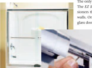
The only tool required is the Allen wrench included in the kit. The EZ Install mounting system relies on turnbuckle-style tensioners that force the top and bottom tracks against the tub walls. Once the frame is up, the towel bars are secured to the glass doors and a bead of caulk is run around the perimeter —
