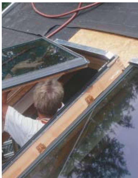
Figure 4. After the carpenters nail down two of the four mounting brackets, they reinstall the sash to make sure that the unit is square (left). Necessary adjustments are made; then the other brackets are nailed off (right).
