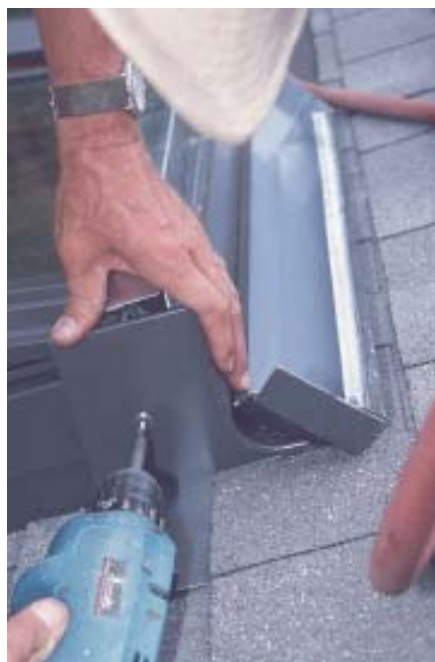
Figure 10. Reinstalling the skylight's cladding completes the process. The bottom goes on first (top left). Slots in the bottom receive the side pieces (top right). Plastic inserts in the sides receive the screws inserted through the head flashing (above left). Finally, the top cladding piece is slipped over the head flashing and secured with two screws (above right).
