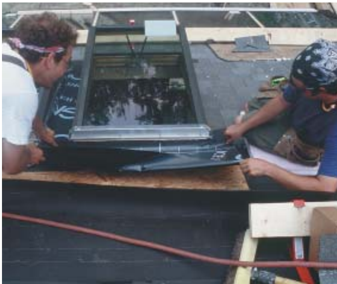
Figure 6. The top piece of membrane laps over the sides (left), and a slit cut outward forms a flap that folds around the corner (right). The membrane's leading edge is adhered to the roof deck under the felt.
