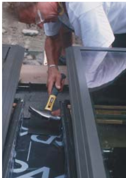
Figure 7. When the shingling reaches the skylight, the sill flashing is slid up from the bottom and fastened at the top corner with the manufacturer's special nails (left). The first piece of step flashing overlaps the sill flashing 3\frac{1}{2} inches. Where adjacent sill flashings overlap, urethane sealant provides extra insurance against leaks (right).
