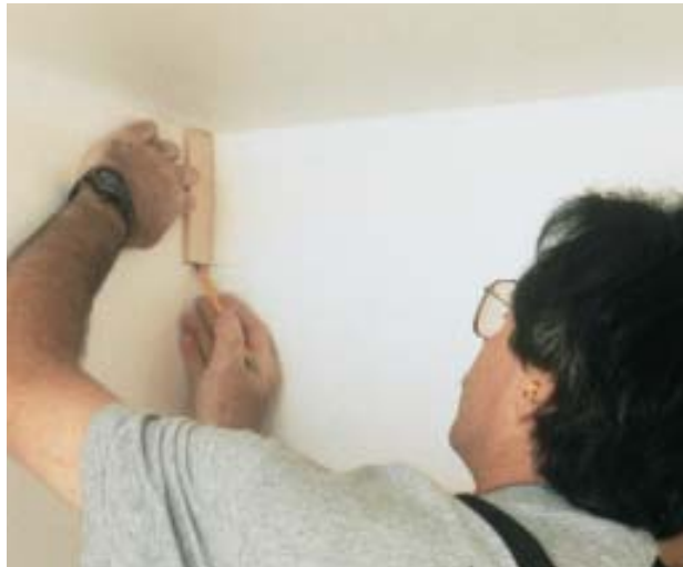
Figure 2. A gauge block the size of the rise simplifies layout.
