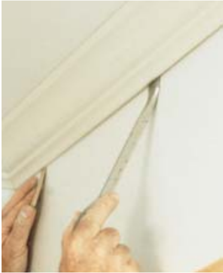
Figure 14. MDF shims are often necessary to close up a joint.
