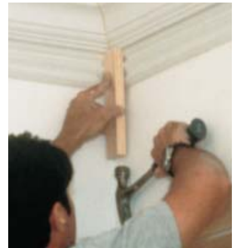
Figure 13. Use a softwood block to drive the corner together, tapping the top of both pieces toward the wall to close a gap at the top of the miter, or tapping up on the bottom edge of the molding to close a gap at the bottom of the miter.
