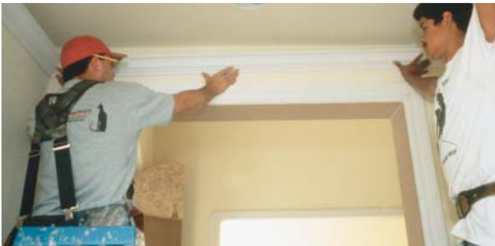
Figure 15. Preassembly guarantees tight-fitting miters, especially with difficult-to-cope dentil crown (above left). (See photo, page 53.) Temporarily secure the corners with miter clamps, then fasten with glue and brad nails (above right). Small hallway and bathroom rectangles should always be preassembled because they can be installed in just minutes (left).
