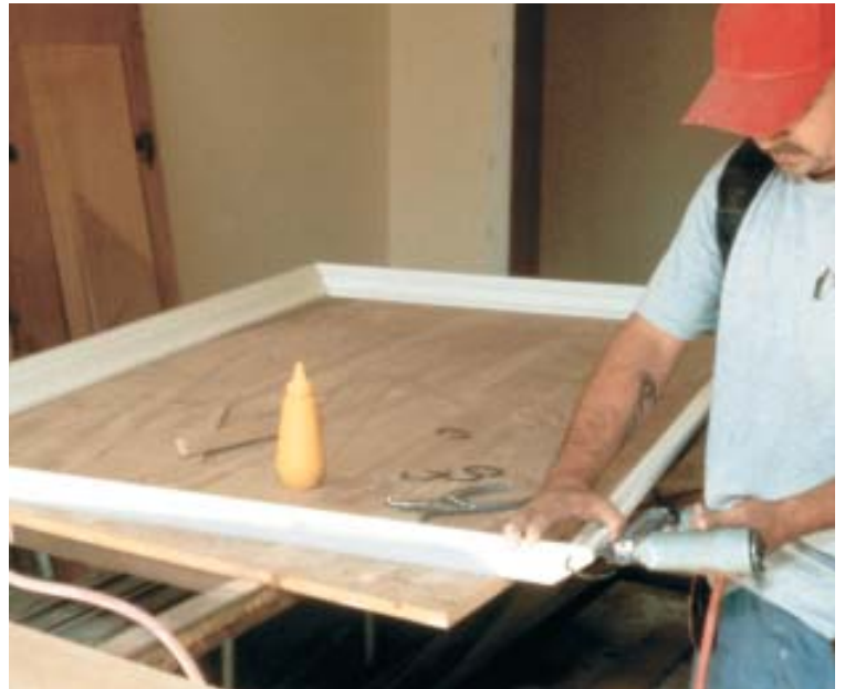
Figure 15. Preassembly guarantees tight-fitting miters, especially with difficult-to-cope dentil crown (above left). (See photo, page 53.) Temporarily secure the corners with miter clamps, then fasten with glue and brad nails (above right). Small hallway and bathroom rectangles should always be preassembled because they can be installed in just minutes (left).
