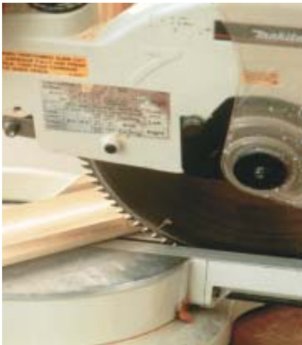
Figure 7. To cut LH inside corners and RH outside corners, the bottom edge must be against the fence and nearly hidden from view, so cut those corners first (top left). Then flip the material, hook your tape on the long point, and make your measurement mark on the bottom edge of the molding (top right). That way you can control exactly where the blade meets the measurement mark (above).
