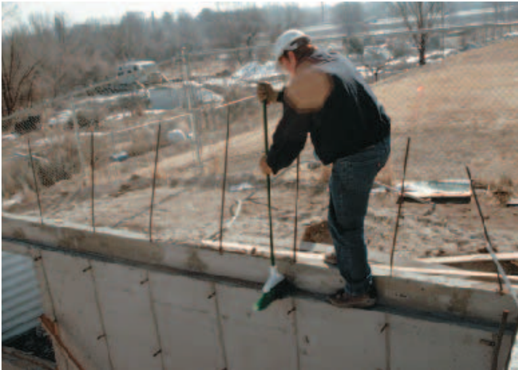
Figure 2. The author set his precast slabs into an 8-inch-deep shelf in the foundation wall. The shelf must provide at least 3 inches of bearing for the precast slabs. Half-inch rebar cast into the foundation wall at 2 inches o.c. will be bent down over the precast sections before the topping slab is poured, to lock the assembly together.
