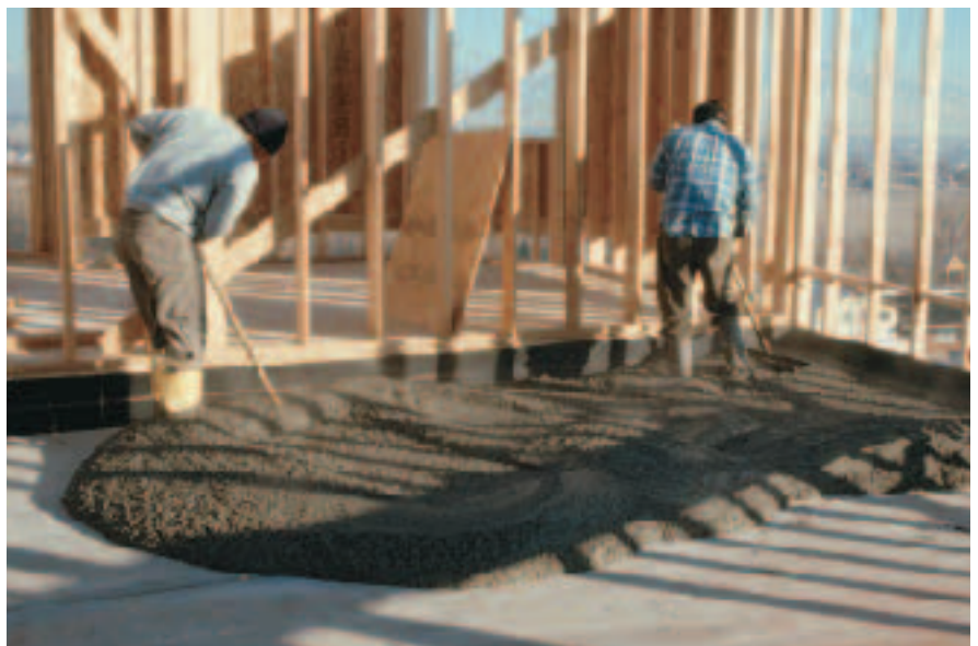
Figure 8. The last step is to pour the concrete topping slab, using a standard 4,000-psi concrete mix.
