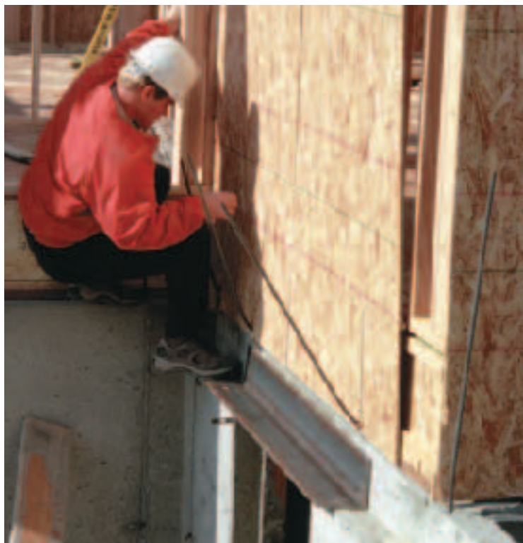
Figure 4. The precast supplier places a 4x4-inch piece of 1/2-inch angle iron over the door opening into the room below the garage. The angle iron will function as a header to carry the edge of the precast slab.
