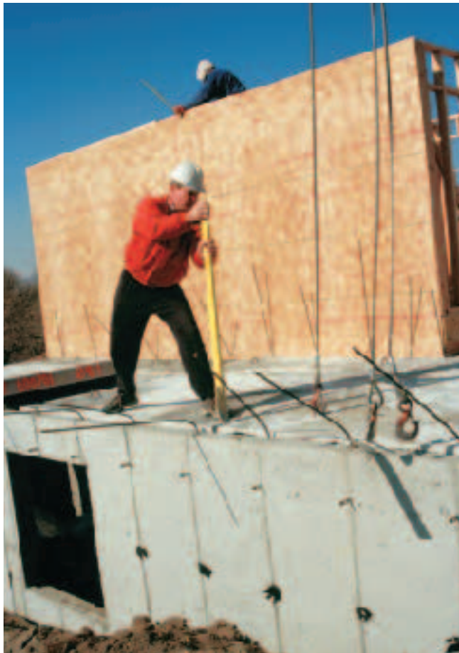
Figure 6. The installer uses a large pry bar to create even spaces between the slab sections. Voids will be injected with foam sealant, then filled with concrete grout.
