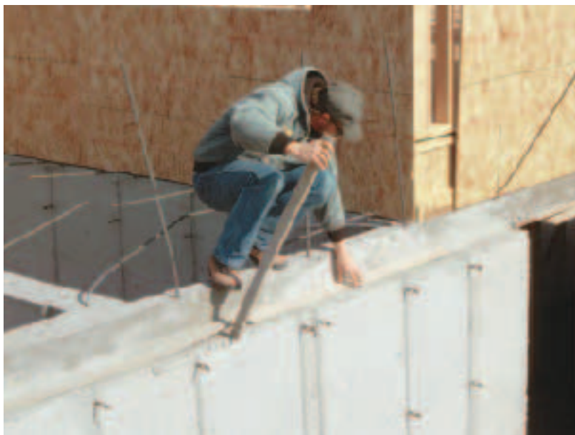
Figure 3. After sweeping the ledge clean, the install crew lays expansion joint material on the shelf around the whole perimeter.
