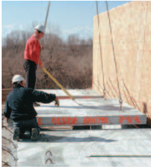
Figure 5. Slab sections are lowered into place by crane. The crane hooks attach to steel cable loops that are cast into the slabs and will be buried in concrete when the topping slab is poured.
