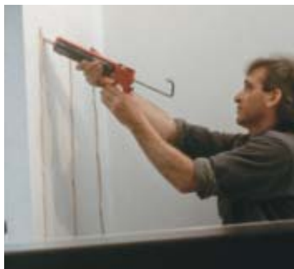
Figure 6. Heavy mirror glass calls for a generous application of special mirror mastic. Drywall substrates must be dust free and sealed for a secure bond.
