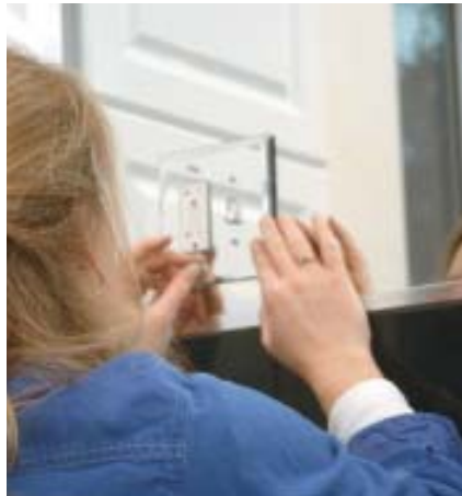
Figure 2. Existing outlets can be incorporated into the mirror field and capped with a reflective cover plate.
