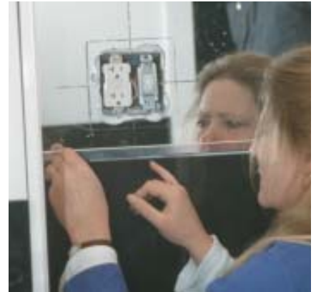
Figure 5. Chrome-plated J-channel supports the mirror until the mastic sets up and hides shims, but also conceals "black edge" corrosion on backsplash-mounted mirrors.
