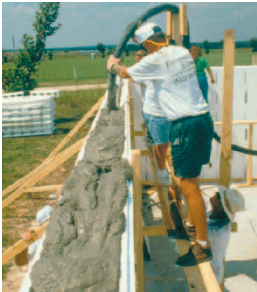
Figure 4. Superplasticizers or mid-range water reducers are often added when concrete needs to be pumped (above). They allow the concrete to flow into the pump (left), reduce wear on the equipment, and ease the job, all while maintaining high quality in the hardened concrete. But it's important to stay on schedule, because if the water reducer wears off while the concrete is still in the pipeline, the machine may bog down, and clearing the pipe can be difficult.
