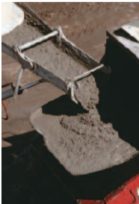
Figure 4. Superplasticizers or mid-range water reducers are often added when concrete needs to be pumped (above). They allow the concrete to flow into the pump (left), reduce wear on the equipment, and ease the job, all while maintaining high quality in the hardened concrete. But it's important to stay on schedule, because if the water reducer wears off while the concrete is still in the pipeline, the machine may bog down, and clearing the pipe can be difficult.
