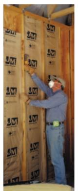
how to insulate the 9-foot walls with 8-foot insulation. Luckily, *Johns Manville* (JM) has released a new 105-inch-long by 15-inch-wide insulation batt. "Installers will love these batts," says John Smith, foam and sheathing market manager for Johns Manville. "This product will help reduce installation time and provide a better fit in 9-foot-high wall cavities." Fewer pieces should mean higher energy efficiency as well.
