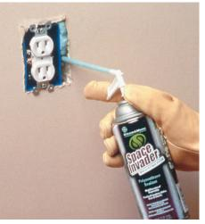
used to plug up all those cracks and gaps in your building envelope. According to GE, the new foam beats the competition in a couple of key ways: It will dispense at any angle — no more standing on your head while foaming. You'll have to work fast, though — Space Invader is
