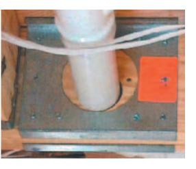
turer cites BOCA and *International One- and Two-Family Dwelling Code* approvals. Check with your code official first. The 2x10 reinforcer allows up to a 6-inch hole to be placed in the center of the joist. Spans and other conditions may restrict the use of the product. The 2x10 joist reinforcer goes for \$8.95.
