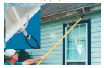
Stubborn debris can be scraped out with the pole or left to dry and blow away. The company has made the downspout removable for cleaning, as well, and that can also be accomplished from the ground. Prices start at \$2.35 per foot including components.
