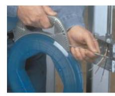
cially suited for conduit runs with multiple bends. Ideal promises that it won't get hung up or deform while in the pipe. The tape is being offered in 50- and 100-foot lengths for under \$100.
