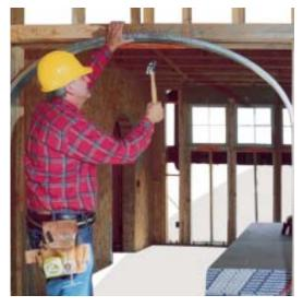
Easy-Arch comes in four different shapes to accommodate the most common curved openings. Quarter and half circles, eyebrows, and ellipses are available in widths from 1/0 to 10/0 for windows, doors, and architectural details. The U-shaped steel channel forms the opening, and wallboard is fastened to the arch's edge. Easy-Arch is lightweight and can be flexed in or out to compensate for a less than perfect opening. The best-selling 3-foot ellipse (TE4-30) lists for under \$30.
