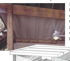
Space, a PVC rain diverter, fits between the deck joists and catches runoff, channeling it to the outside edge of the deck or a gutter system. F-brackets mounted on the side of the joists secure the panels without restricting seasonal
