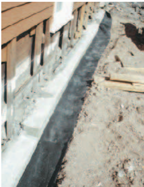
Figure 6. The topmost edge of the membrane was left loose for two months to allow the backfill to settle (right). After being cut and fitted over stepped sections of the foundation, it was covered by galvanized flashing that was later tucked beneath the siding (below).
