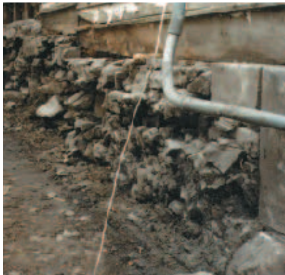
Figure 1. The existing rubble foundation was sitting on well-drained soil and supported the building adequately, but it was far too rough to accept the waterproofing membrane needed to deflect heavy spring runoff.
