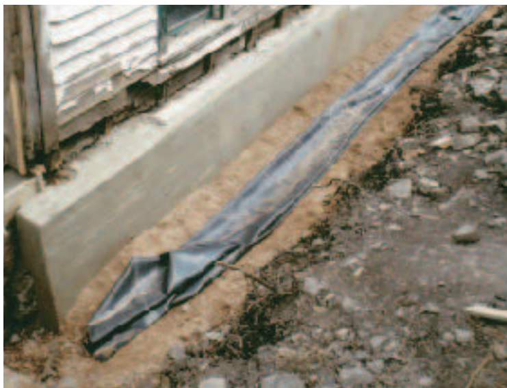
Figure 4. The new poured wall locked the rubble in place and provided a smooth surface for a waterproofing membrane. A smooth layer of roadbed material in the bottom of the trench helps protect the membrane from punctures.
