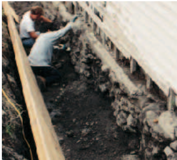
Figure 2. Wall forms were made from 2x4s and full sheets of \frac{3}{4} -inch plywood. Before they were secured to the wall in preparation for the concrete pour, the forms were leaned back against the side of the trench to help keep dirt out of the excavation while the existing walls were being cleaned.
