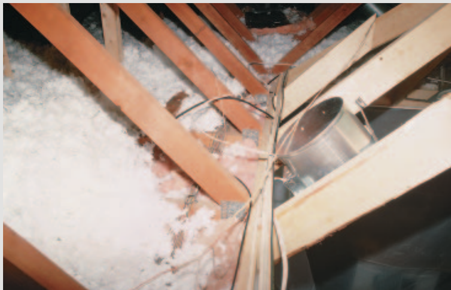
Figure 3. Cutting the bottom chord of the truss a little beyond the metal plate allowed the original truss web to provide some support for the drywall ceiling.
