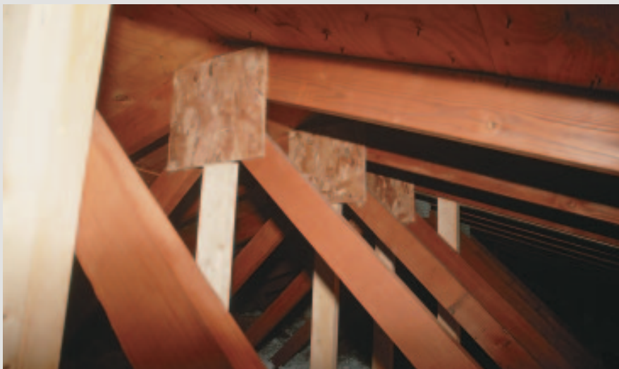
Figure 1. The first step in modifying the truss roof structure (top) was to add support posts from the peak to a bearing wall below (bottom). OSB gusset plates secured the connection.
