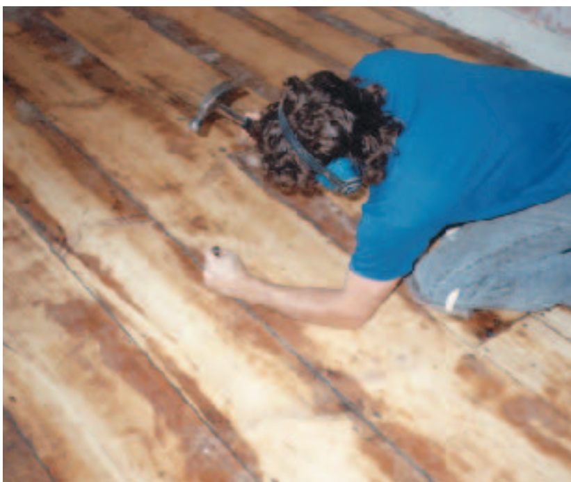
Figure 2. All nails need to be countersunk before any fine sanding takes place. If the drum sander hits a nail, it will groove the sandpaper and cause a disfiguring “nail run.”
