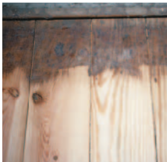
Figure 3. A first rough cut with the drum sander using coarse grit can pull off linoleum and its adhesive but may not expose the wood in low spots (left). The drum sander also leaves an unsanded area near the walls (above), which has to be sanded with the edger.
