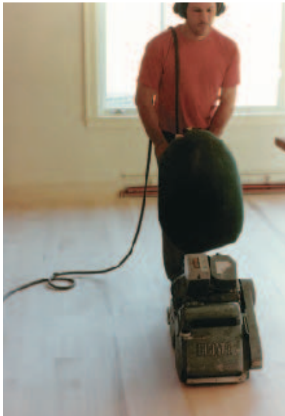
Figure 4. Straight cuts parallel to the boards using grits as fine as 80 create a flat, smooth surface that will accept stain. It's important to wear hearing protection and to keep the power cord out of the way of the machine.
