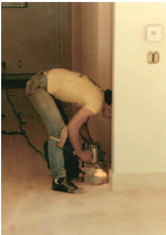
Figure 5. When operating the edger, the author rests his elbows on his knees to reduce the strain on his back. The edger is moved in a circular motion.
