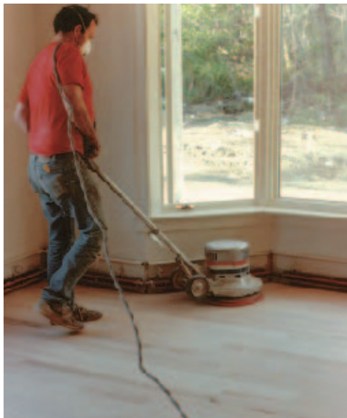
Figure 6. The buffer sits on a synthetic fiber pad and a sanding screen and sands with a circular motion. The whole screen should contact the floor as evenly as possible to create a uniform scratch pattern with no visible swirls. An 80-grit or, at most, 100-grit screen should be used to leave the wood rough enough to absorb stain and finish.
