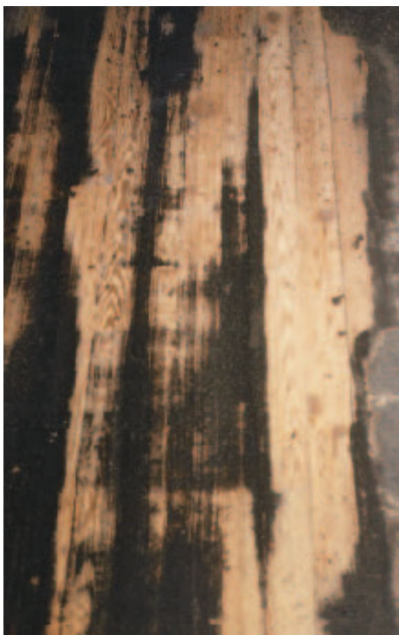
Figure 3. A first rough cut with the drum sander using coarse grit can pull off linoleum and its adhesive but may not expose the wood in low spots (left). The drum sander also leaves an unsanded area near the walls (above), which has to be sanded with the edger.
